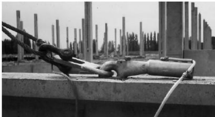
Shape 2.3: Round-headed transport anchor
