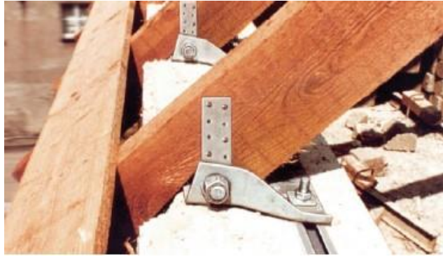
Shape 3.3: Application on rafter shoe
