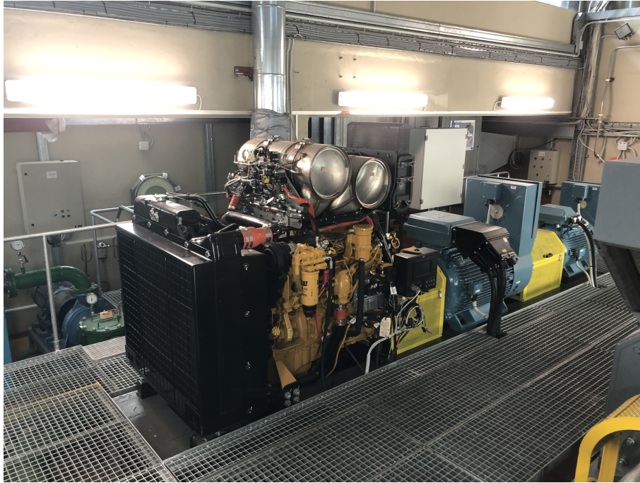
Figure 1.3: Placement of all units on the common bedplate.
