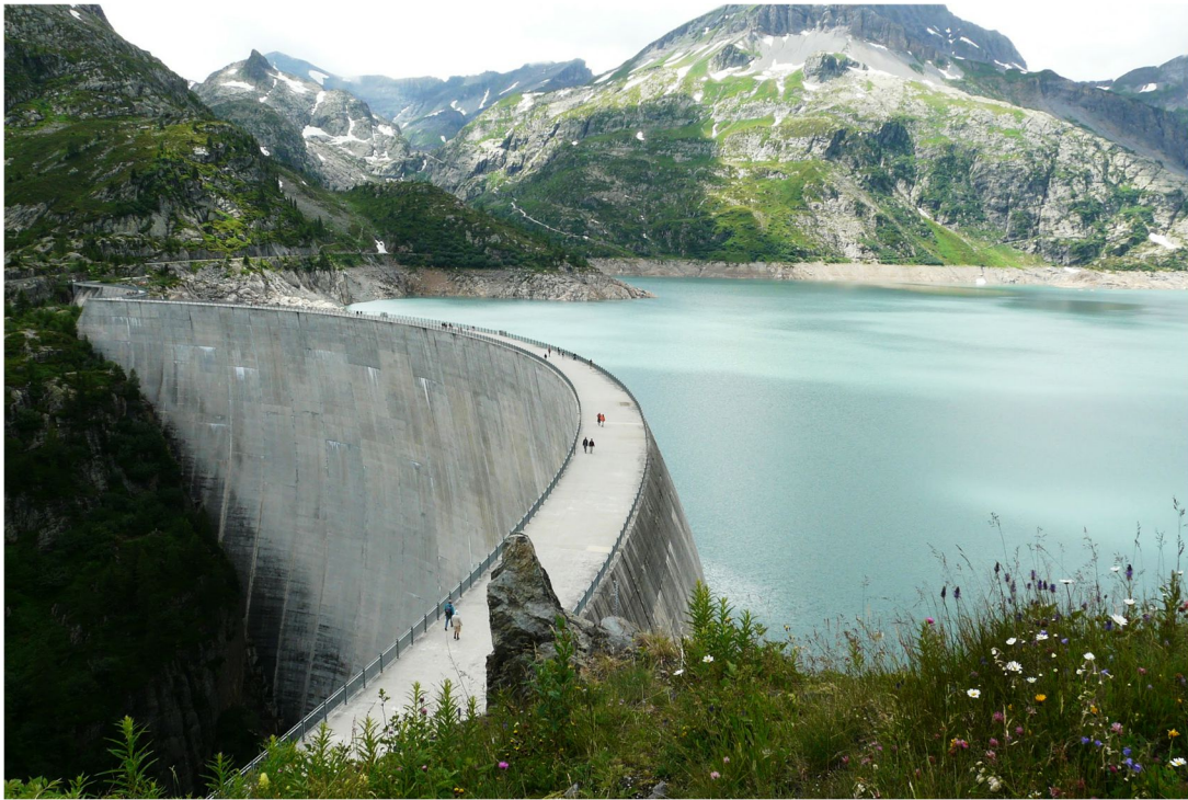
Figure 21. Example of arched dam of architectural and landscape significance – Barnerine or Emosson dam (Switzerland): Image source: https://lh5.googleusercontent.com/p/AF1QipMuEgKJDDHwrsHSEFol7il51mzR2GAAL2-3fgxJ=h1440
