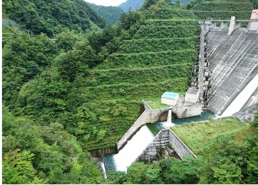
Figure 25. Example of dam with restored excavation slopes – Fukushima dam (Japan). Image source: https://lh5.googleusercontent.com/p/AF1QipN8v9YgphbIHZA_A_S2kFEMImwiksyMkRvOoq_=h720
