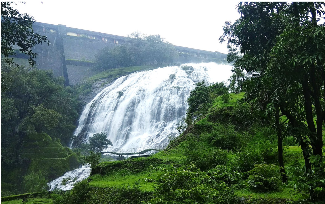
Figure 22. Example of dam with non-standard landscape design of outlet works - Bhandardara or Wilson (India) with overflow of outlet water on rocky dam abutments. Image source: Error! Hyperlink reference not valid.
