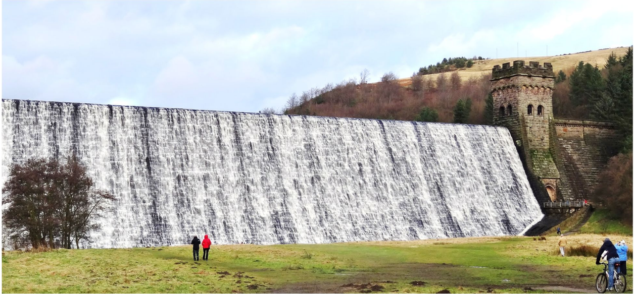
Figure 23. Example of dam with a special architectural design of its spillway with overflow over dam body – Derwent dam (UK). Image source: https://lh5.googleusercontent.com/p/AF1QipNV_vl6wBhjacsDsgQLuWEC EL2h-UkFP7v_3Mc2E=w1280-h720-pd
