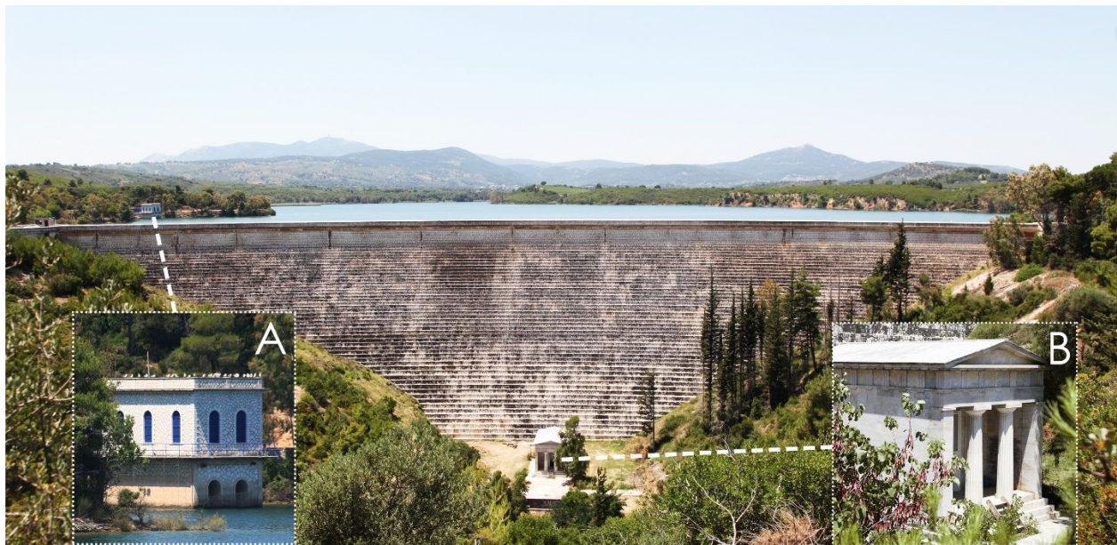
Figure 8. Example of architecturally designed dam (Marathon dam in Greece). Picture of the downstream face of the dam, which is overlaid with marble from the mine of Penteli that was also used to build the Temple of Parthenon, including pictures of architecturally designed appurtenant structures: (A) water intake tower, with similar design with the downstream face of the dam and (B) reservoir control building at the base of the dam, built to resemble the ancient temple-like structure called Thesaurus (treasure) and built after the victorious battle of Marathon (480 BCE) in Delphi. The new building was given this form in order to symbolize the victory of modern Athens in the battle against water scarcity. The dam of Marathon is not a hydroelectric dam but is indicative of the architectural adaptability of dams and their appurtenant structures, that can, and has been utilized in hundreds of hydroelectric dams internationally. Technical information on Marathon dam can be found in Soulis et al. (Soulis et al., 2019).
