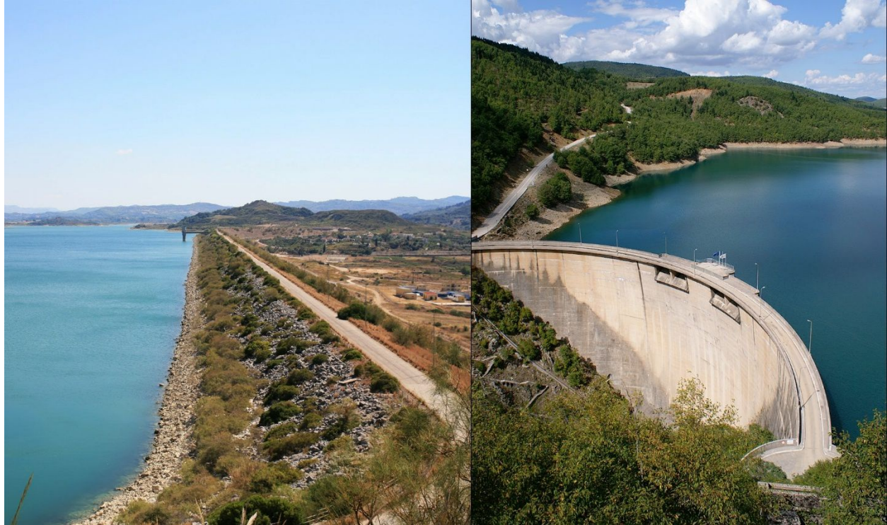
Figure 28. Photographs of Pinios (left) and Plastiras/Tavropos dam (right) 17 .
