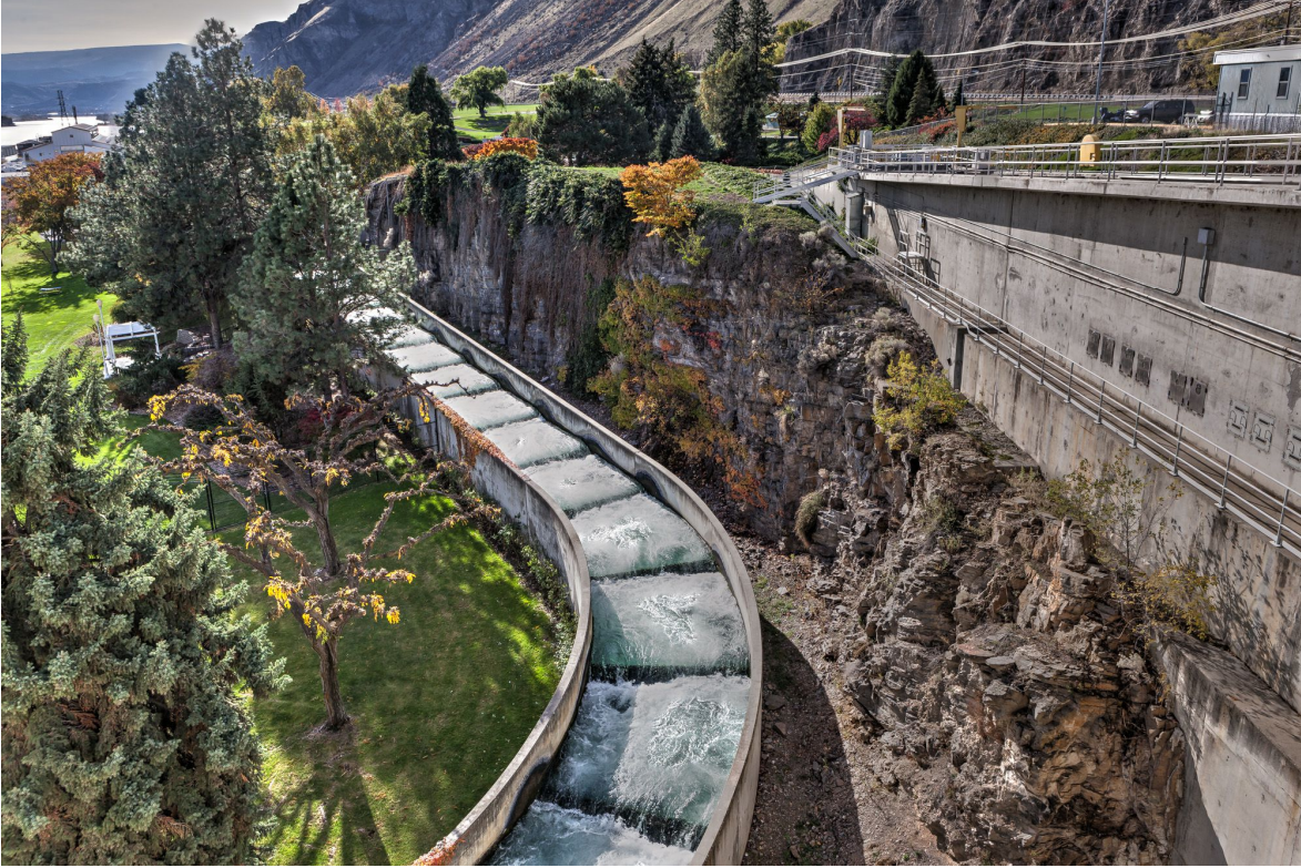
Figure 24. Example of dam with landscape design of appurtenant structure, in this case of fish pass, - Rocky Reach dam (USA). https://lh5.googleusercontent.com/p/AF1QipP5I8DvzPQGwtKryb0t7UbOCAKI3UYkWI74 30_w=h1440
