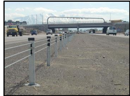
Cable median barrier
