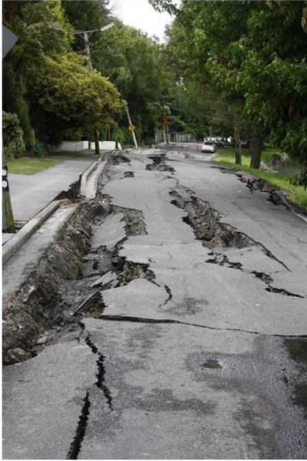
Figure 1.1: Liquefaction-related phenomena during major earthquakes. (a) Bearing capacity failure of shallow foundations, (b) floating of light structures, (c) ground failure due to lateral spreading, (d) soil ejecta of the liquefied soil to the ground surface and (e) sinking of heavy objects.
