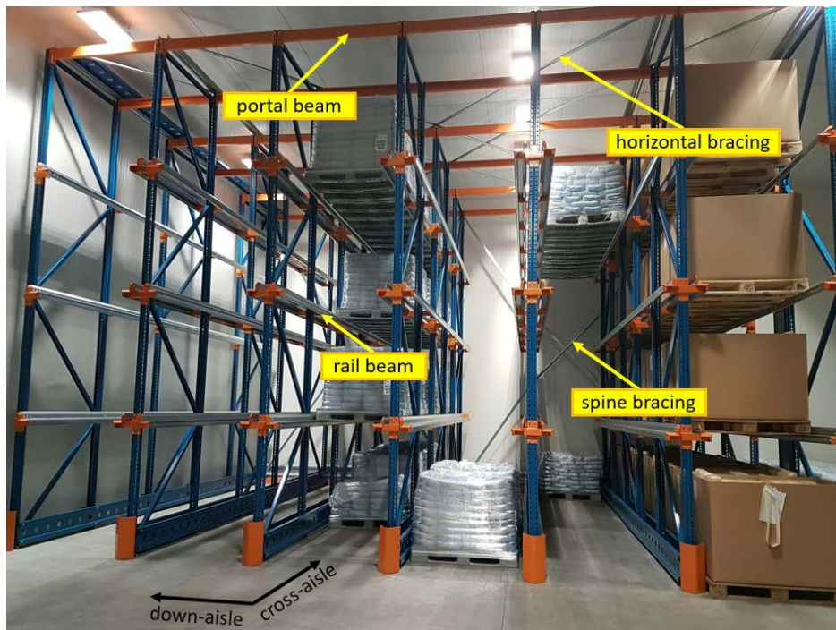
Figure 2.3: Primary structural components of a drive-in steel racking system. In drive-in racks, the forklifts enter inside the rack in order to deposit and withdraw the pallets (photo courtesy of Nedcon B.V.).
