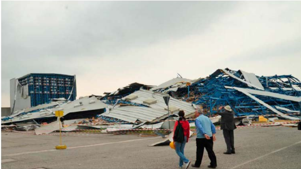
Figure 1.4: Collapse of Ceramic Storage warehouse in Sant' Agostino due to 2012 Emilia-Romagna earthquake, Italy (Kanyilmaz et al., 2016).
