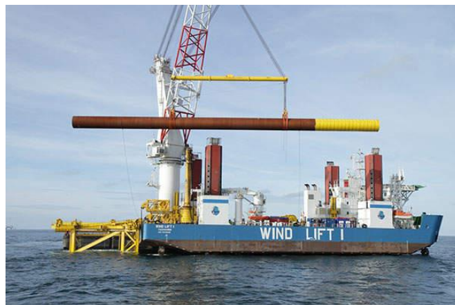
Figure 2-34 Piles being installed at the Bard Offshore 1 Wind Farm ( www.power-technology.com )
