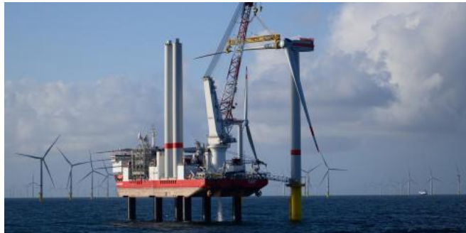
Figure 2-11 Blade installation at the Borkum Riffgrund II Offshore Wind Farm ( www.jandenul.com )
