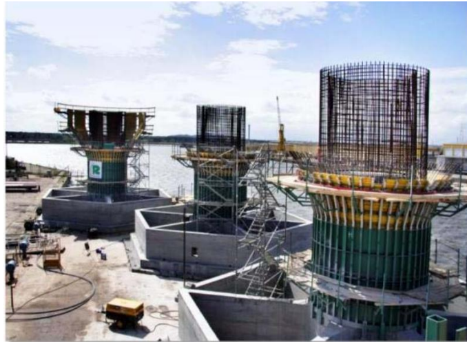
Figure 2-37 Concrete foundations being cast (Jeppsson, Larsen, & Larsson, 2008)
