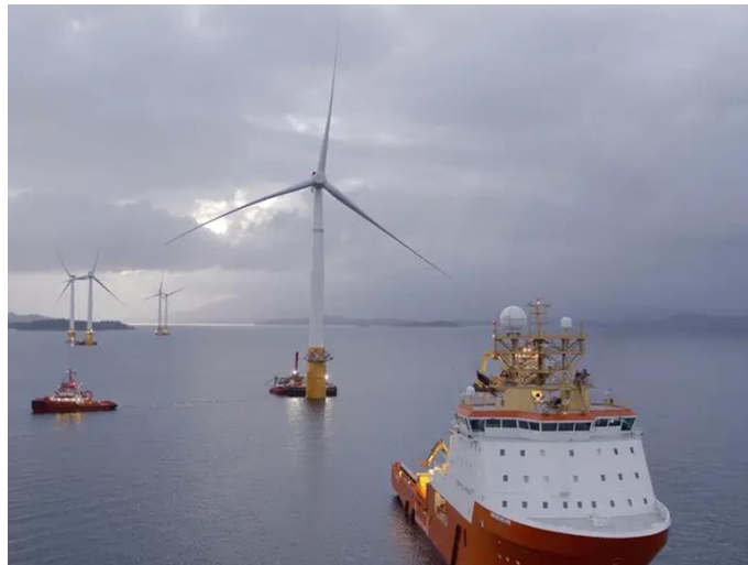
Figure 2-50 Assembled structures being towed to the project's site (www.businessinsider.com)
