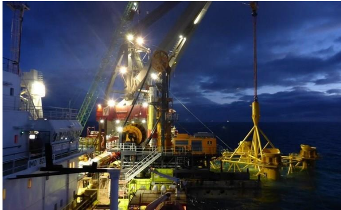
Figure 2-15 Pre-piling template being installed for the Beatrice Offshore Wind Farm (renews.biz)
