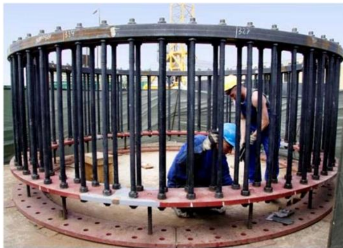
Figure 2-38 Tower bolts to be cast into the foundation (Jeppsson, Larsen, & Larsson, 2008)
