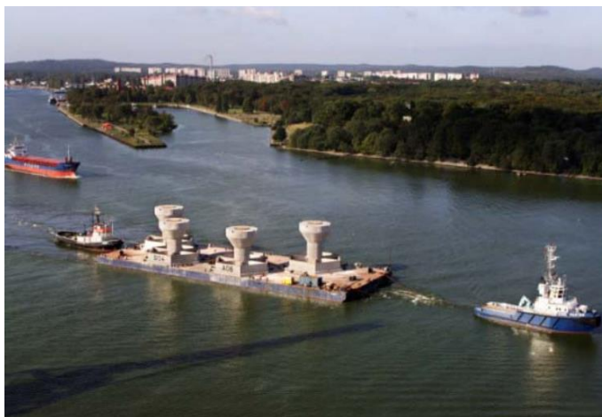
Figure 2-39 Concrete foundations being towed to Lillgrund site (Jeppsson, Larsen, & Larsson, 2008)
