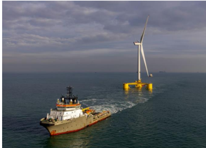
Figure 2-44 Kincardine Offshore Wind Farm assembled units being towed to project site ( www.offshorewind.biz )
