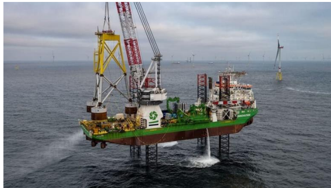
Figure 2-24 Suction bucket jacket being installed by heavy lift jack-up vessel ( www.mynewsdesk.com )
