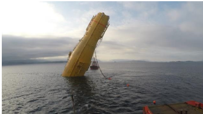
Figure 2-47 Spar buoys being upended ( www.ptil.no )
