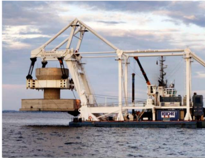
Figure 2-40 Concrete substructures being lowered into position (Jeppsson, Larsen, & Larsson, 2008)
