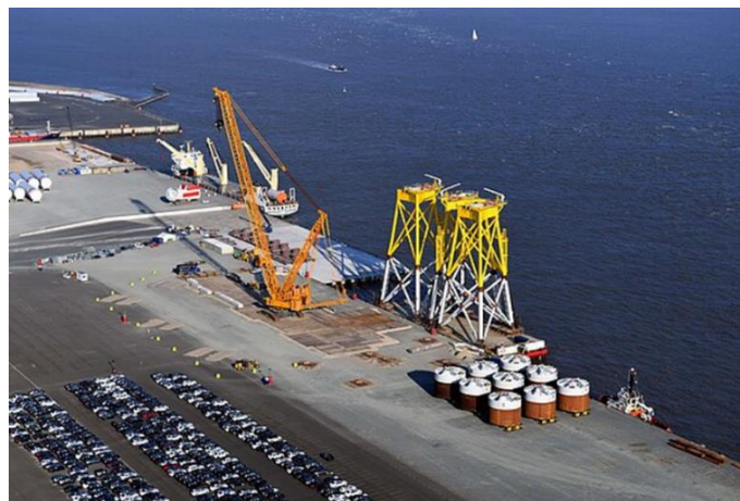
Figure 2-22 Borkum Riffgrund II Offshore Wind Farm jackets and suction buckets at the assembly terminal (www.rhenus.group)
