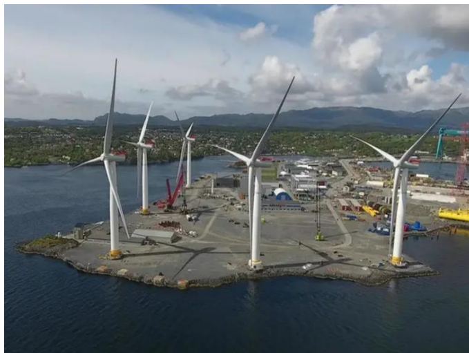
Figure 2-48 Turbines being assembled at project's assembly base ( www.businessinsider.com )
