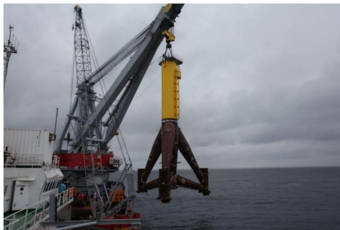
Figure 2-29 Borkum West II Offshore Wind Farm tripod being installed (www.trianel-borkum.de)
