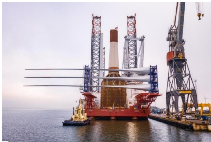
Figure 2-53 Mono-bucket substructure and turbine components being loaded onto jack-up vessel ( www.offshorewind.biz )
