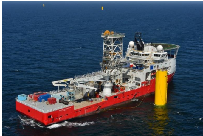
Figure 2-30 Borkum West II Offshore Wind Farm tripod fully installed ( www.trianel-borkum.de )
