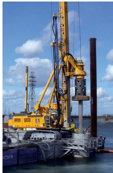
Figure 2-9 Seabed drilling rig ( www.bauer.de )
