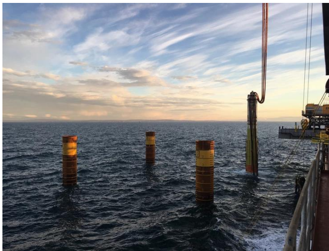
Figure 2-16 Piles being installed for the Beatrice Offshore Wind Farm (www.beatricewind.com)
