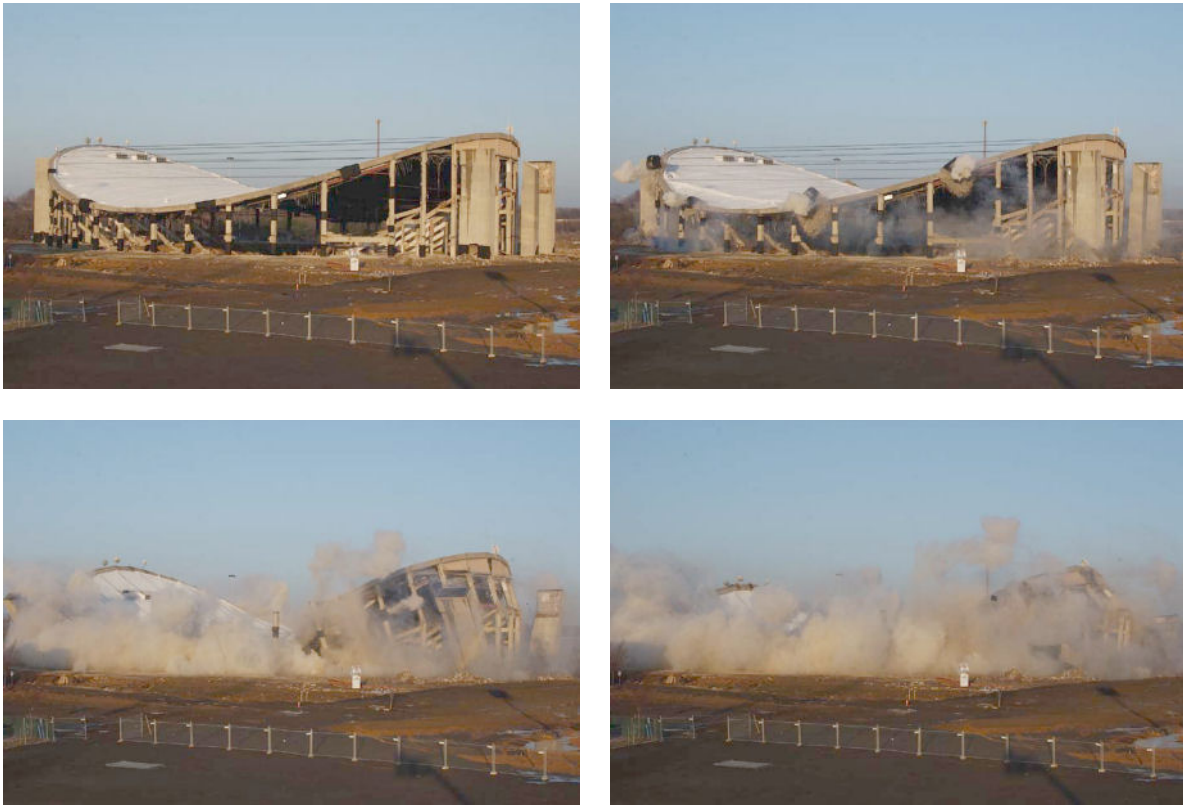
Photo 1-6: US Air Arena in Largo, Maryland, U.S.A. during its demolition in 2002
