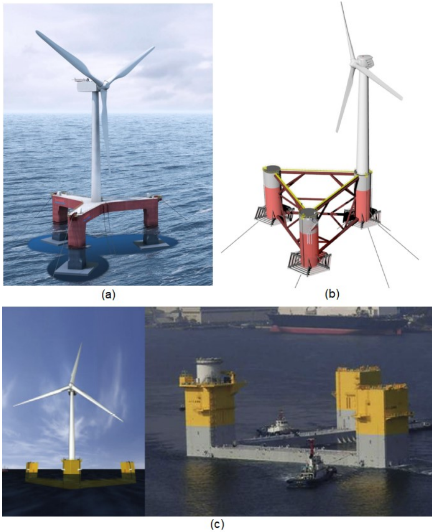
Figure 1.3: Floating platform concepts: (a) GustoMSC Tri-Floater, (b) WindFloat and (c) V-shaped braceless semi-submersible. Source: Respective literature.
