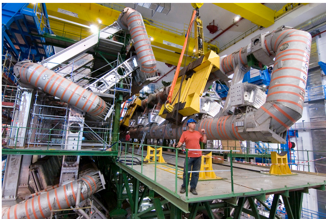
Figure 2.4: ATLAS Barrel toroid magnet during the installation of one torus.
