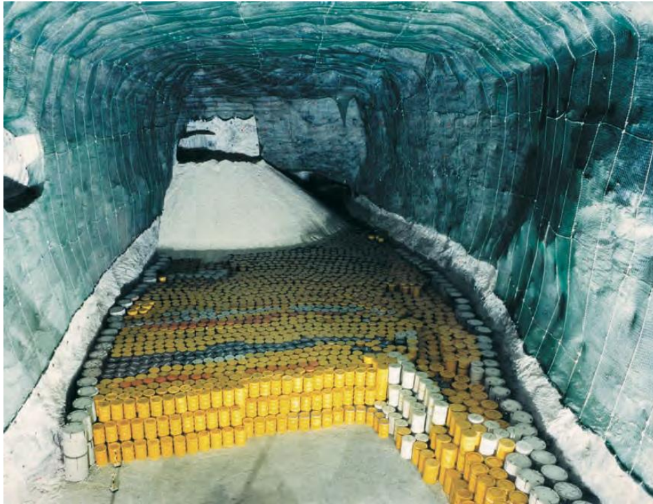
Figure 9 Underground Radioactive Waste Disposal in Morsleben (Germany) in rock salt (Source: Benardos, Lecture Notes).
