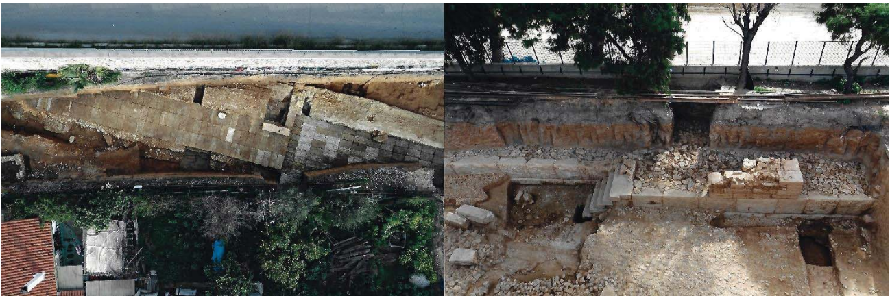
Figure 1: EFAPN Findings of the Southern Long Wall below the surface metro tracks. Photo from the archive of EFAPN.
