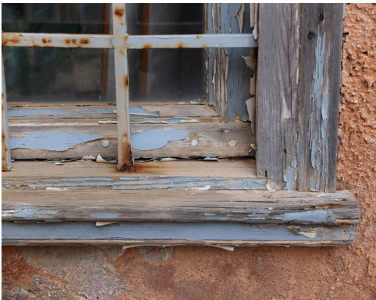
FIG. 18.8 Water damage and signs of corrosion to the windows of a restored building in the LTCP, 2017.
