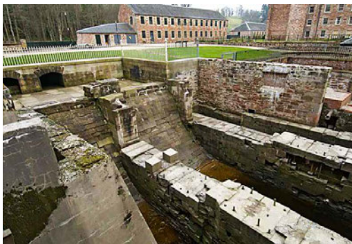
FIG. 3.3 The excavated waterwheel pits (Historic Environment Scotland).
