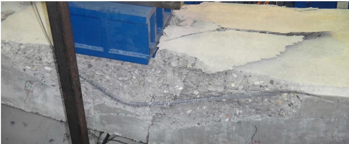
Fig. 5.28- S4- Buckling of rebars at the end of the test (fig. 5.30 and 5.31, points D and D')
