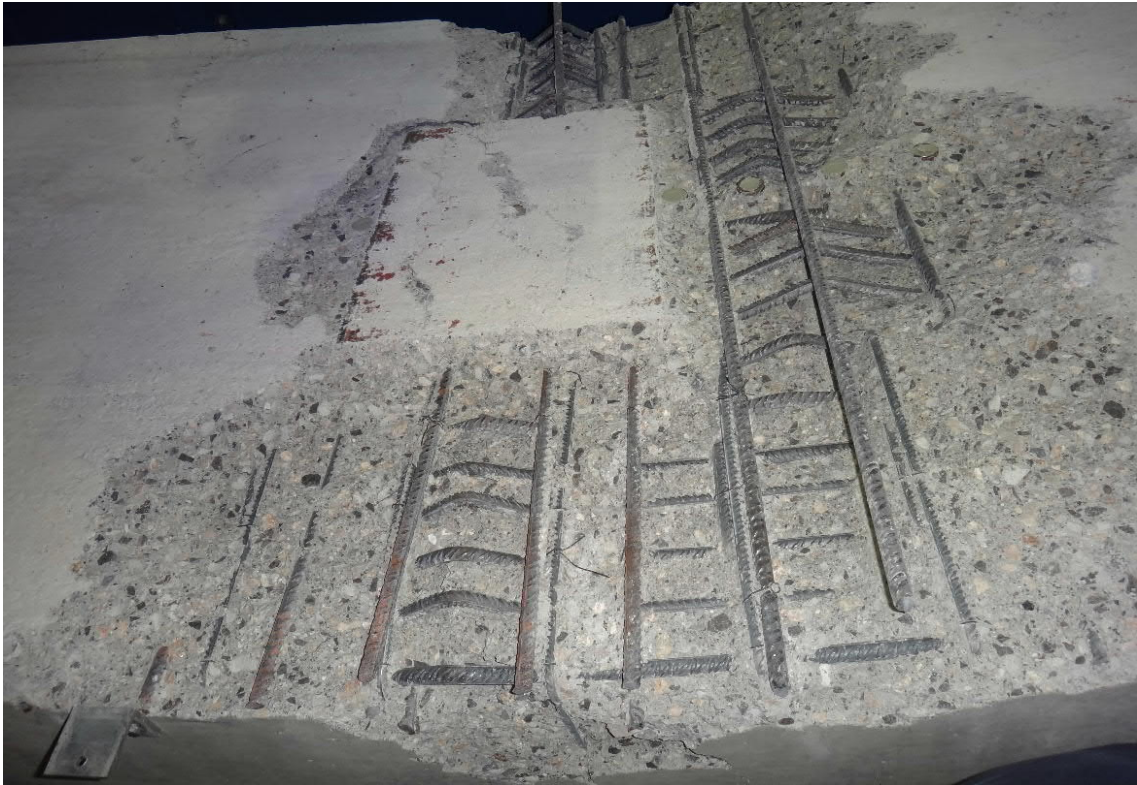
Fig. 5.102- S6a- The beam after the removal of loose concrete
