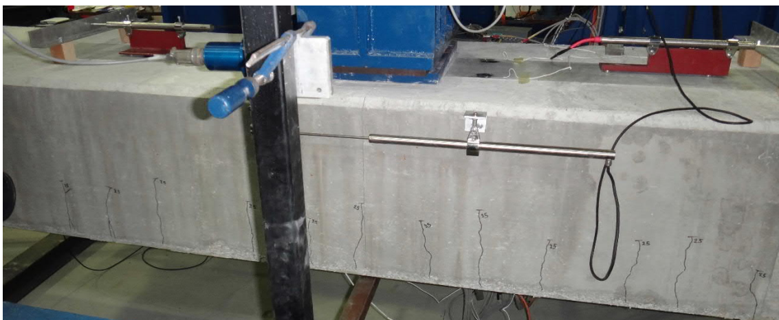
Fig. 5.65- S11- Cracks at deflection of 25 mm (fig. 5.71 and 5.72, points B and B')
