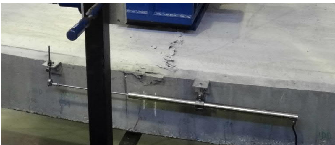
Fig. 5.97- S6a- Cracks at the top face of concrete (fig. 5.104 and 5.105, points C and C')
