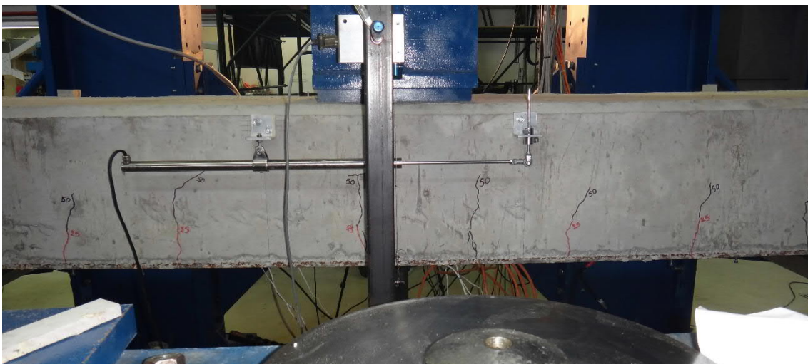
Fig. 5.37- S5- Cracks at deflection of 50 mm (fig. 5.42 and 5.43, points B and B')
