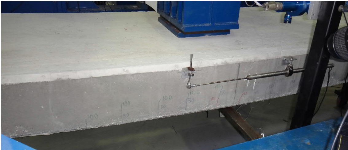
Fig. 5.96- S6a- Cracks at deflection of 100mm (fig. 5.104 and 5.105, points C and C')
