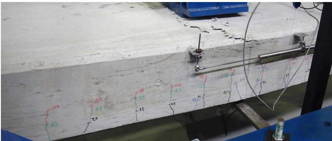
Fig. 5.126- S7- Cracks at deflection of 150 mm (fig. 5.130, point E)
