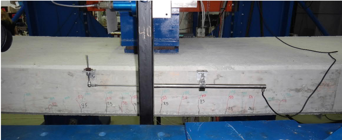
Fig. 5.112- S6b- Cracks at deflection of 100 mm (fig. 5.117 and 5.118, points C and C')
