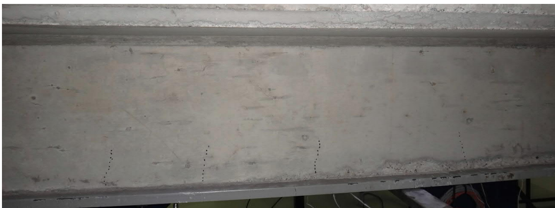
Fig. 5.152- S9- Hair-line cracks at deflection of 19 mm (fig. 5.159 and 5.160, points A and A')
