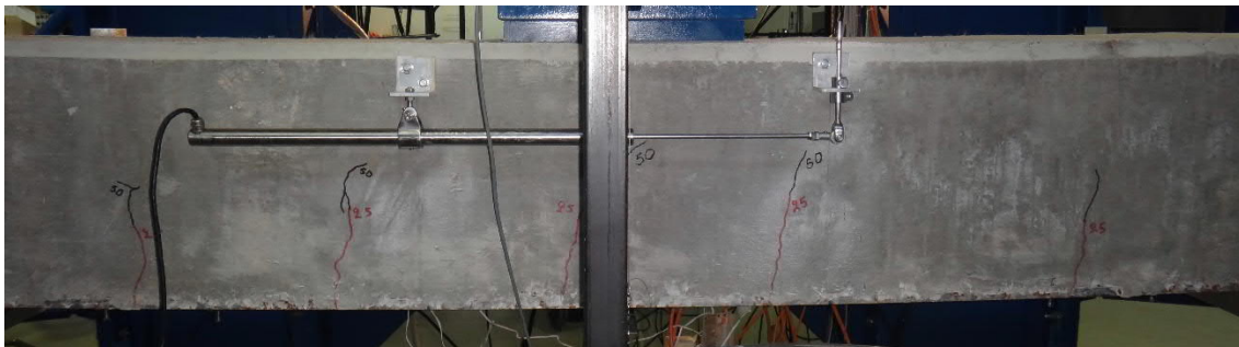
Fig. 5.25- S4- Cracks at deflection of 50 mm (fig. 5.30 and 5.31, points B and B')
