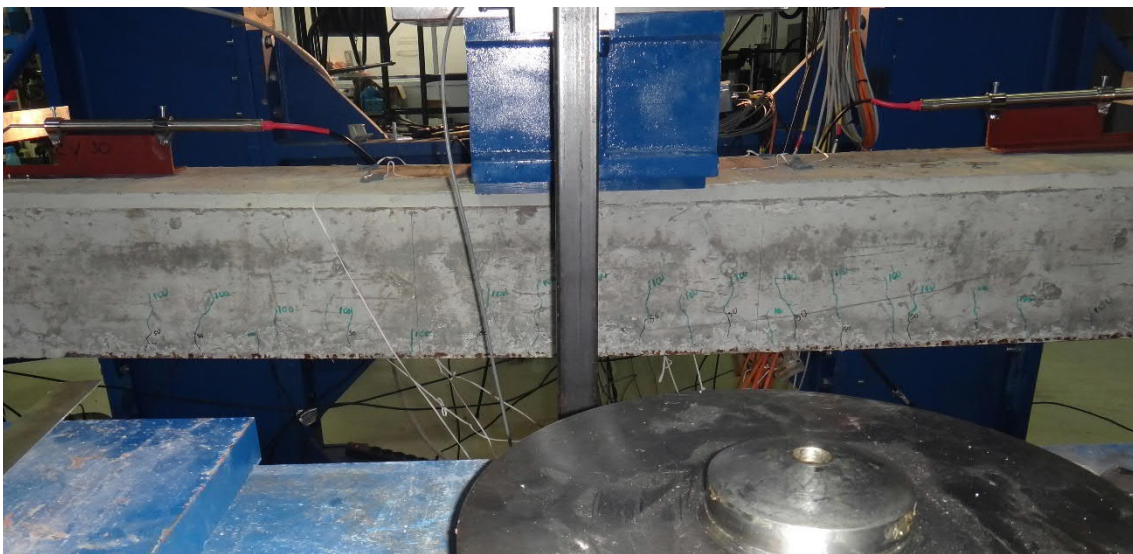
Fig. 5.80- S12- Cracks at deflection of 100 mm (fig. 5.85 and 5.86, points C and C')
