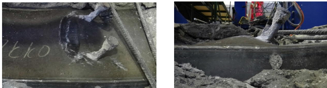
Fig. 5.5- S2- Buckling of the top plate
