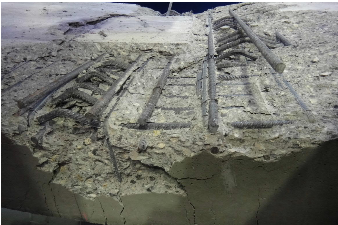
Fig. 5.103- S6a- The beam after the removal of loose concrete
