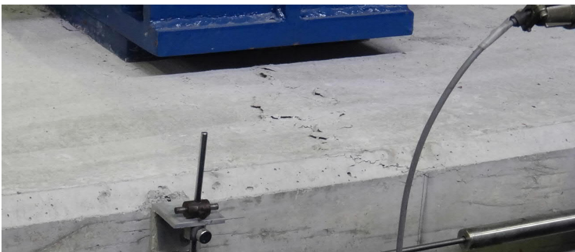
Fig. 5.127- S7- Cracks at the top face of concrete (fig. 5.130, point D)
