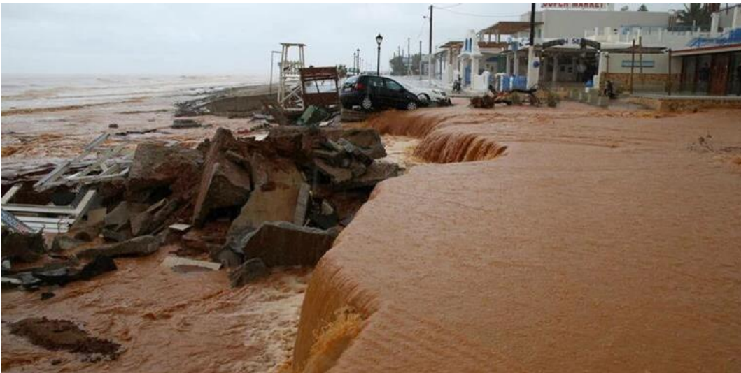
Figure 1-3 Damages of coastal infrastructures and intense beach erosion due to high energetic storm events; Crete, Greece 2013.
