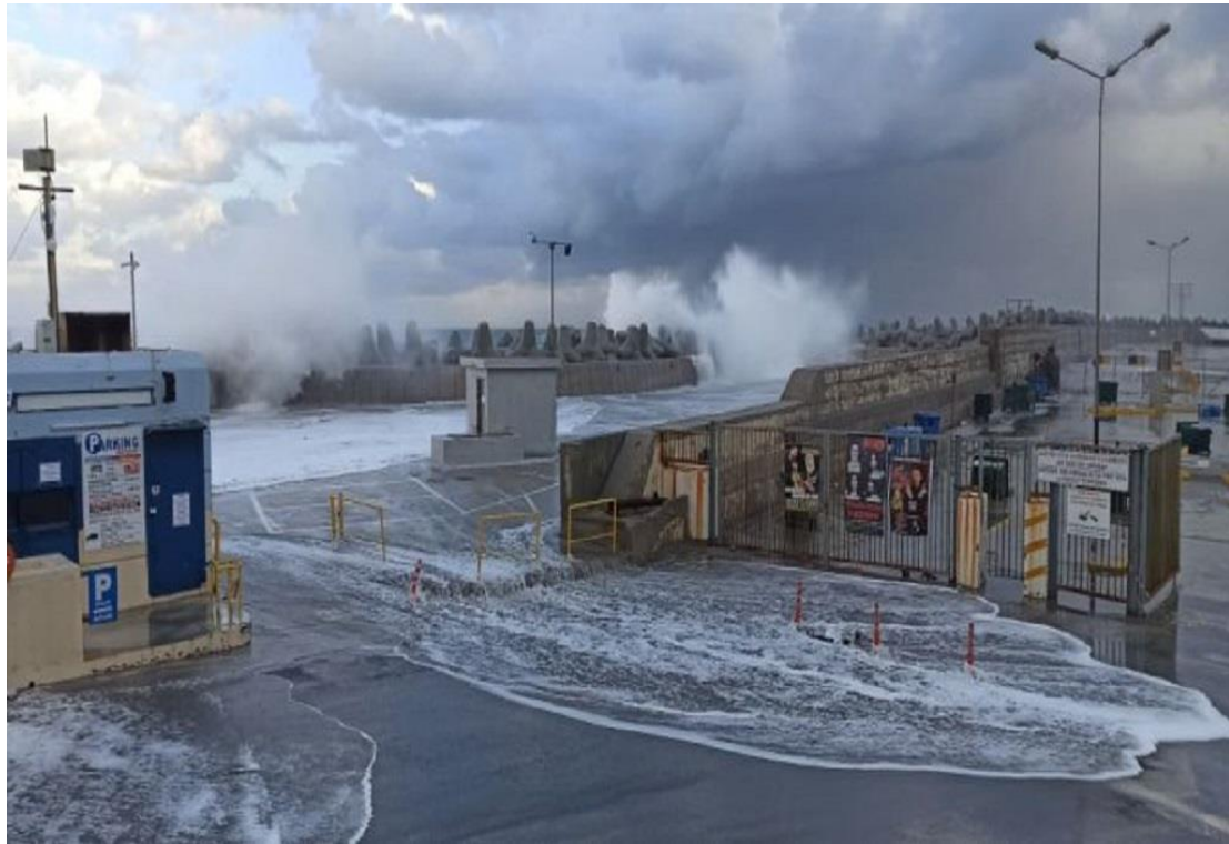
Figure 2-3 Recent floods at the harbour area of Rethymno (2019).
