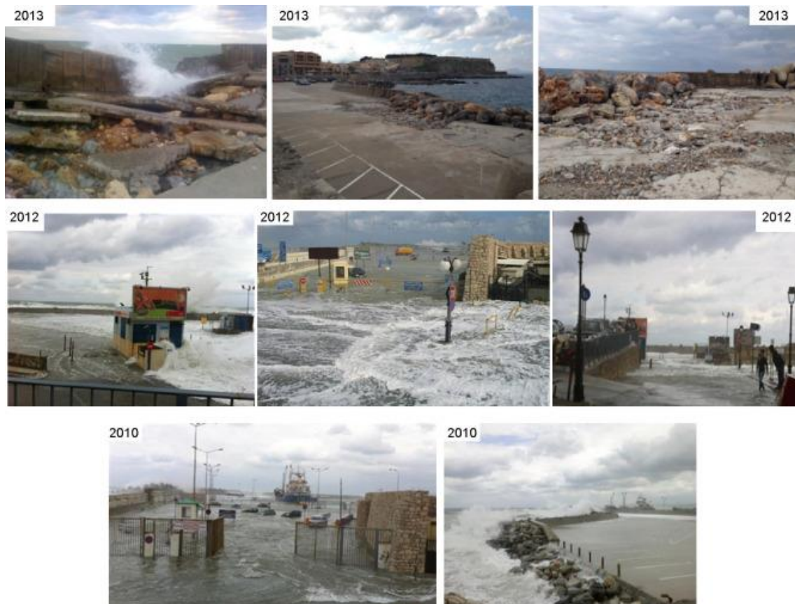
Figure 2-2 Recent floods at the harbour area of Rethymno (2010–2013).
