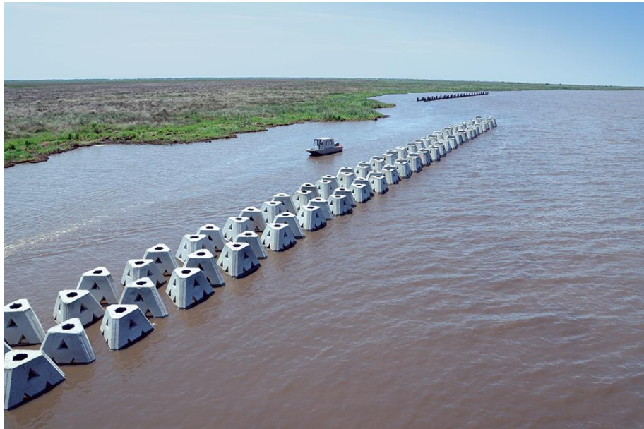
Figure 1-8 Artificial Reefs & Coastal Restoration Inc.'s patented Wave Attenuation Device. (Source NPCA and Living Shoreline Solutions Inc).
