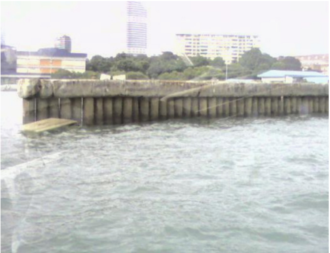
Figure 1.3: A bottom-sitting, surface-piercing pile breakwater along the coast of Singapore [2]
