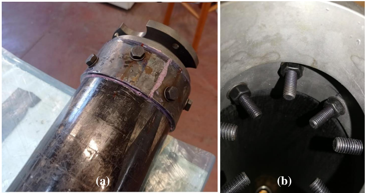
Figure 4.2 (a) External view of the edges of the shaft where attached metal ring-shaped piece and the bolts are visible (b) Internal view of bolts penetration in the shaft-flange connection
