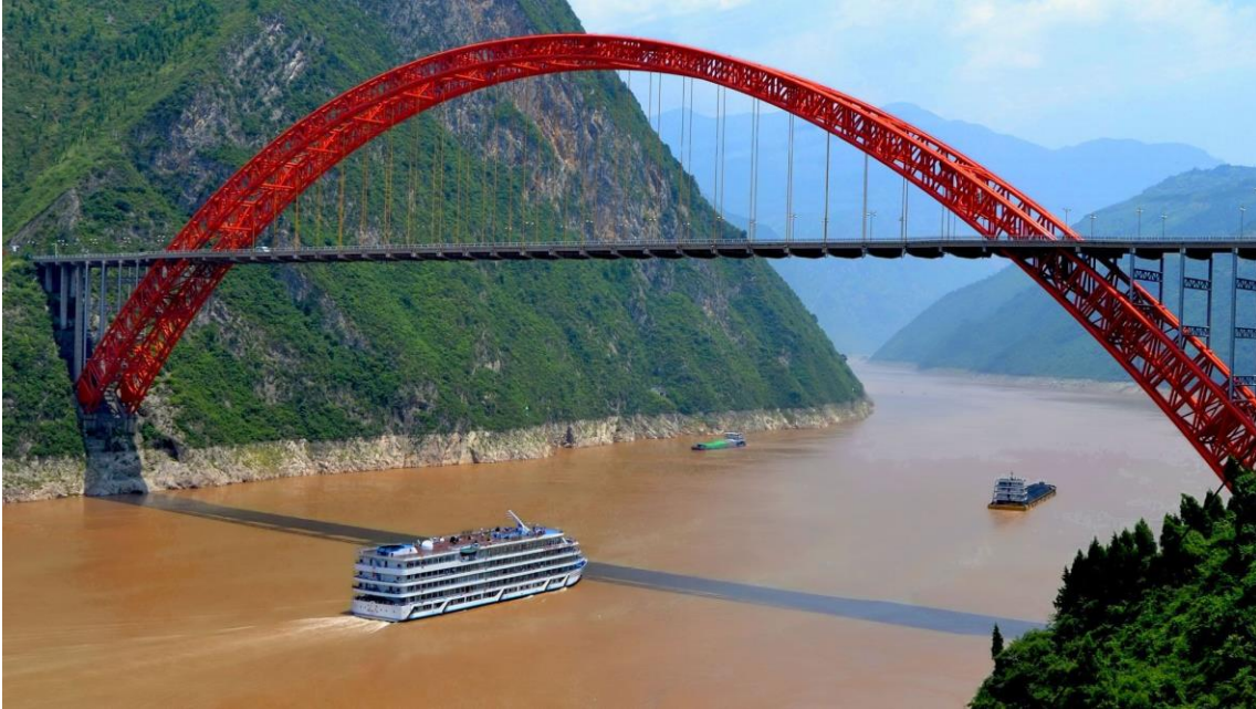
Σχήμα 1.2 : Wuxia Yangtze River Half Through Arch Bridge, China
