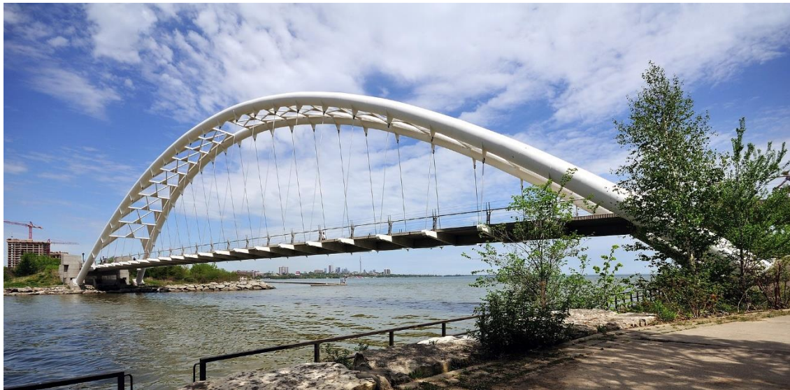
Σχήμα 1.3 : Humber Bay Through Arch Bridge, Ontario Lake
