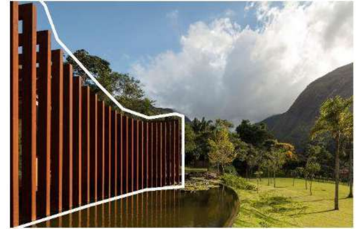
Εικ.49: Nascimento Chapel by Miguel Pinto Guimarães A' design award and competition 2019 πηγή: https://competition.adesignaward.com/design.php?ID=80733 >, ίδια επεξεργασία
