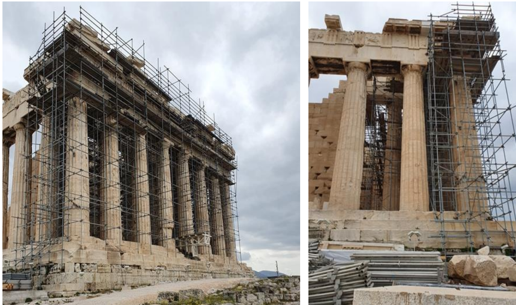
Figure 31: (left and right) Restoration works of the Opisthonaos (2021)
