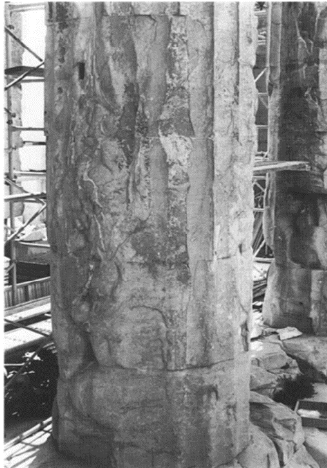
Figure 48: The first four drums of column O.K 3 with newer fillings in their fractures (Study for the restoration of the Parthenon, K. Zambas, vol.3b, YSMA 1994)
