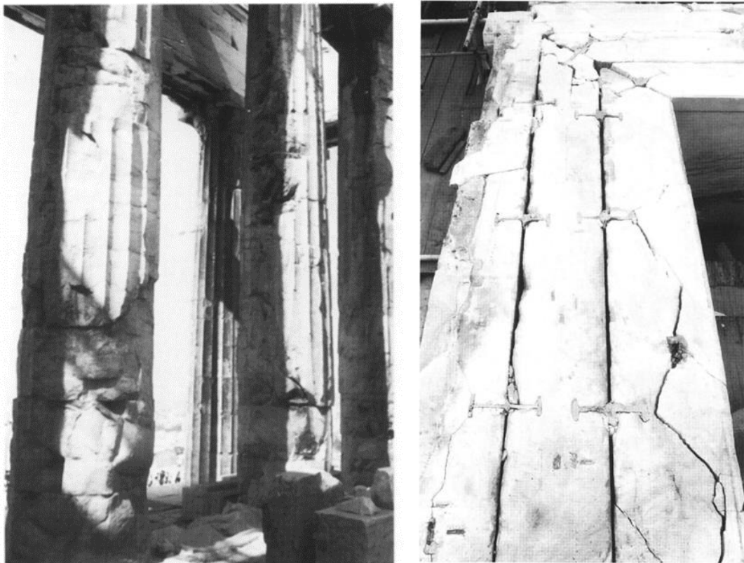
Figure 37: (left) Columns of Opisthonaos, (right) Epistyle block of SW side of the Parthenon with extensive fracturing at the joints (Study for the restoration of the Parthenon, K. Zambas, vol.3b, YSMA 1994)
