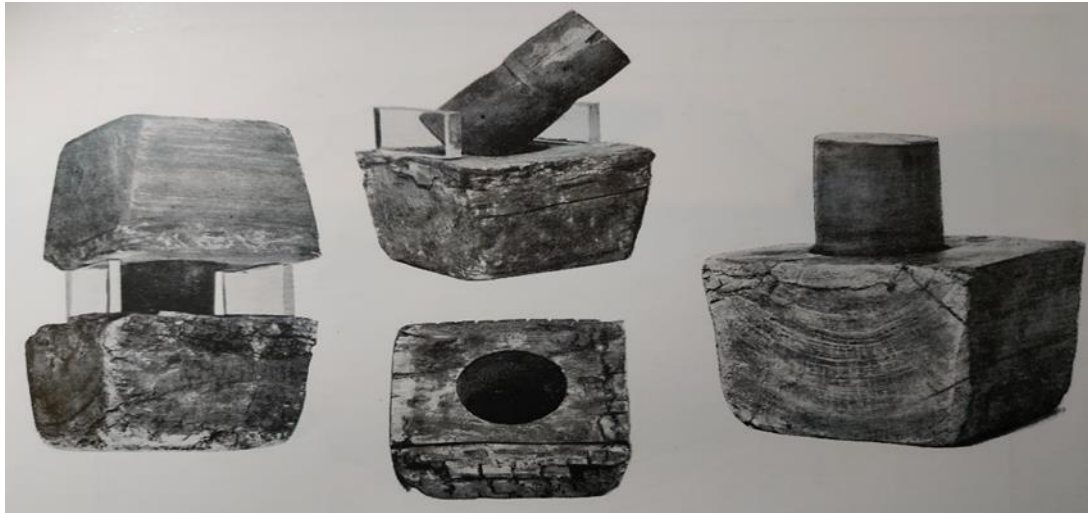
Figure 16: Poles and empolia ( The Architecture of the Parthenon , A. K. Orlandos, vol. B, The Archaeological Society at Athens , Athens 1977, fig. 100)
