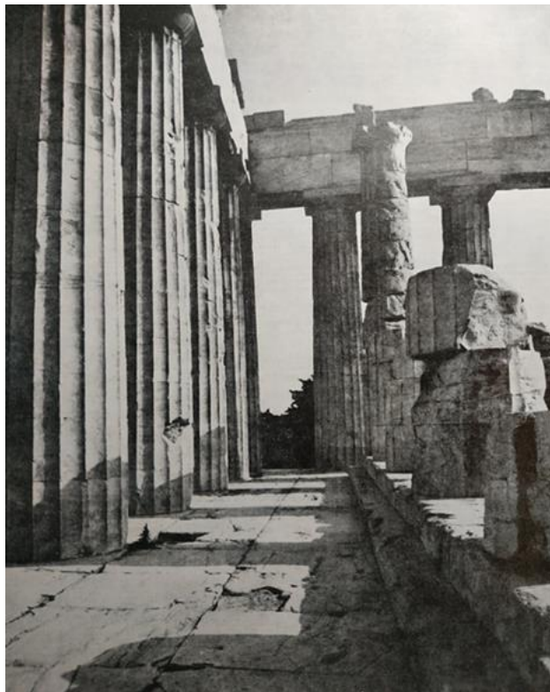
Figure 28: A view of the columns of the pronaos with the restored SE column in the background. On the left is the east side of the peristyle, with the wide east pteron extending between the two. (The Architecture of the Parthenon, A. K. Orlandos, vol. B, The Archaeological Society at Athens, Athens 1977, fig. 195)
