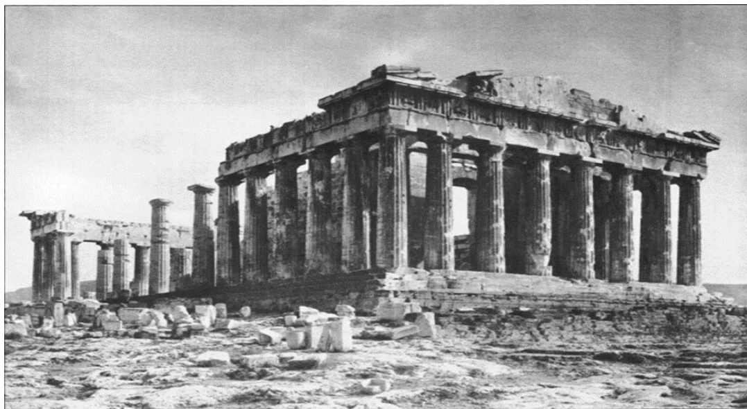
Figure 49: The Parthenon from NW after the restoration of 1844. Fully restored columns 9 and 11 and partially restored columns 6, 7, 8 and 10 are visible. (Study for the structural restoration of the northern side of the Parthenon, K. Zambas, YSMA 2002)
