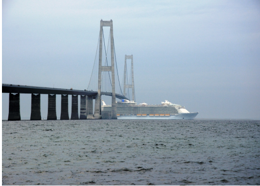
(a) M/V Allure of the Seas, passing under the Great Belt Bridge (2010)
