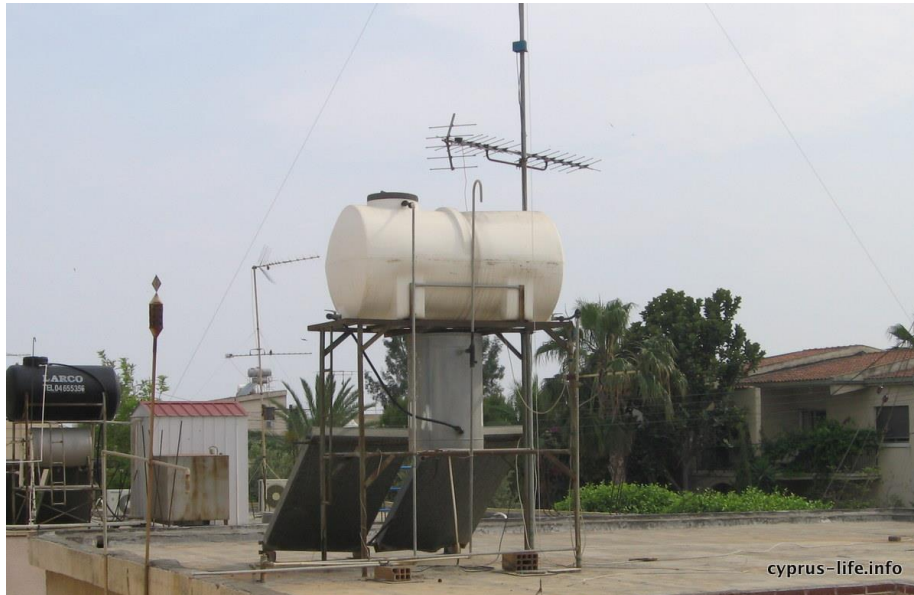
Figure 2.2 Typical water tank on the roof of a building in Cyprus [23]
