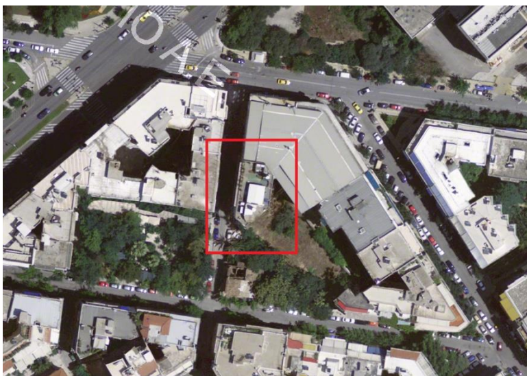
Figure 140. Orthophoto of the case-study area at the scale of 1:1000. The studied building is located within the red rectangle.
