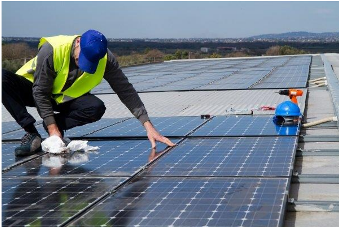
Image3.12: P/V system maintenance [3.20]
