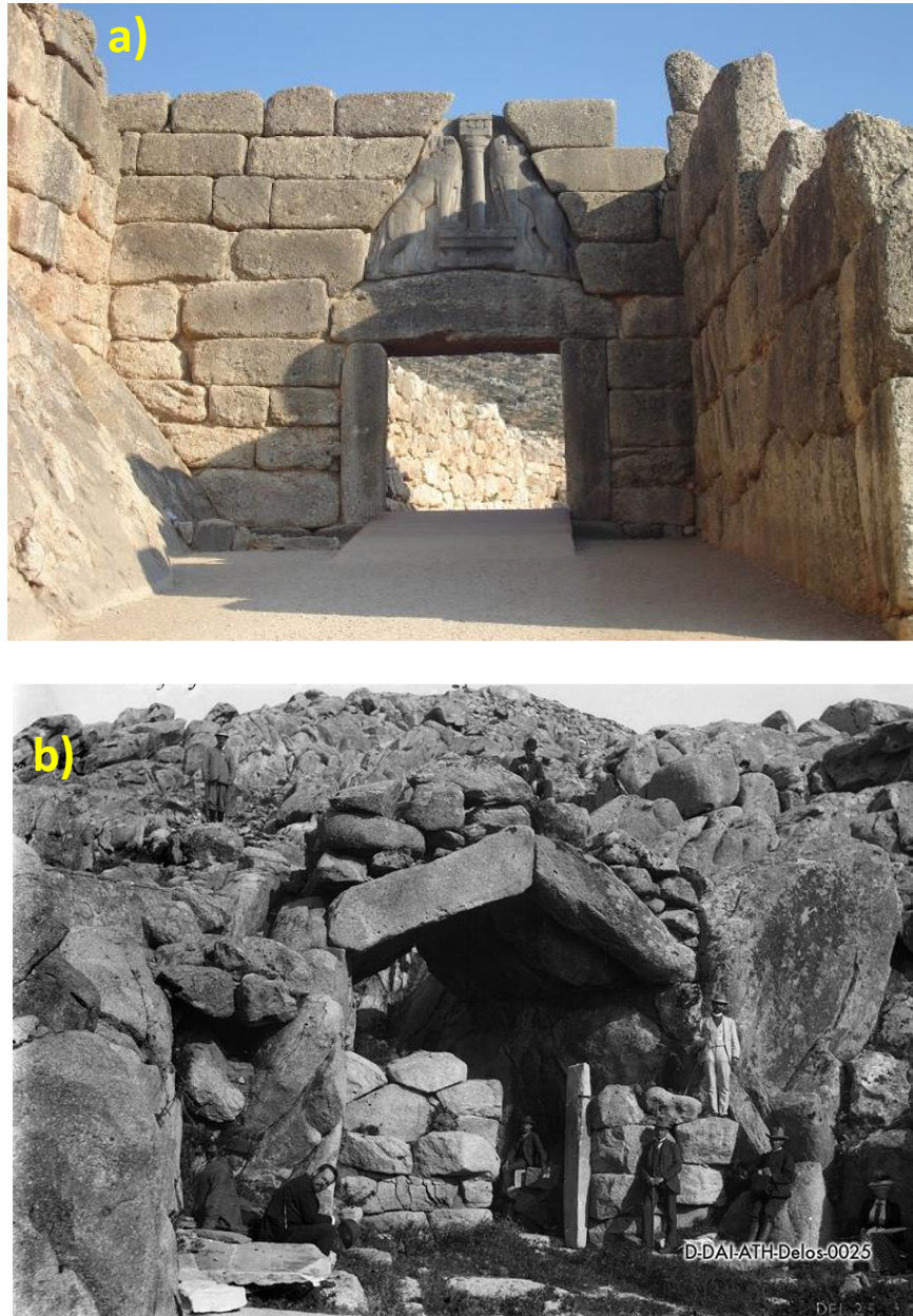
Figure 2.1 Examples of a post and lintel system (a- the Lion Gate at Mycenae) and a false arch (b- the sanctuary of Hercules in Delos).
