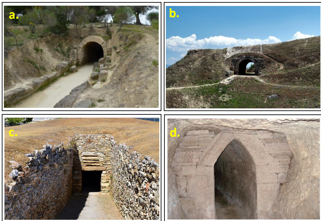
Figure 1.5 Geo-structures of antiquity: (a) vaulted tunnel at the Entrance of Nemea stadium, (b) vaulted tunnel at the Entrance of Sikyon Theatre, (c) tholos tomb in Acharnes, and (d) bored tunnels at the Eupalinian aqueduct.
