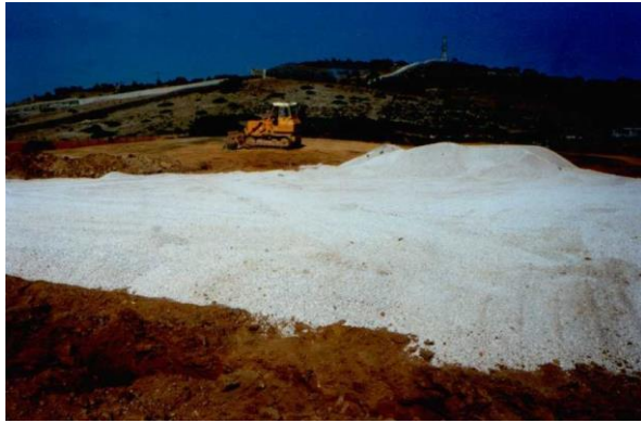
Photo 12. HDPE Cover. First layer, 30 cm of fine gravel as capillary barrier.
