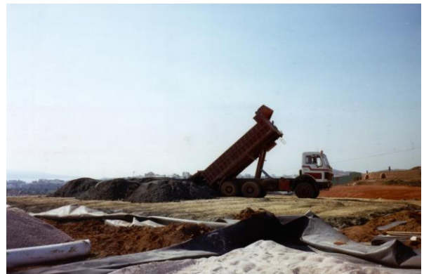
Photos 19. The deposition of Bodosakis pyrites at the Kavodokanos test area.
