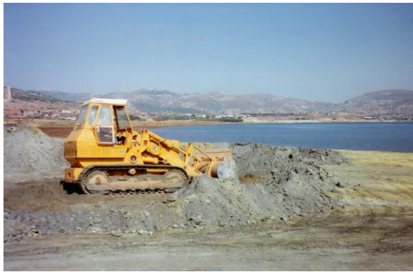
Photo 18. The excavation of Bodossakis pyrites from Thoricos bay.
