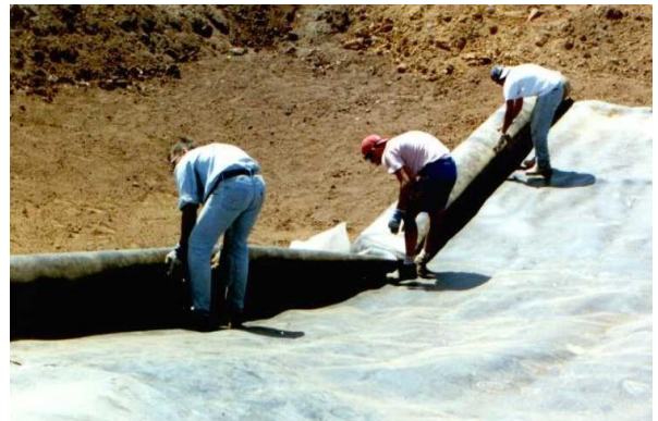
Photo 10. Installation of the lysimeters (left) and the geomembrane (right).
