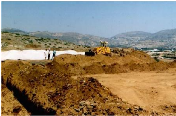
Photo 9. Installation of vertical geomembrane liners for the isolation of test plot areas.
