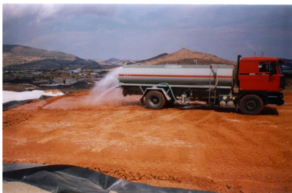
Photo 16 . Compacted Clay Cover. Watering of the clay layer.
