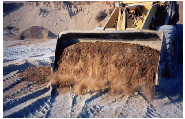
Photo 32. Laying down of compost.
