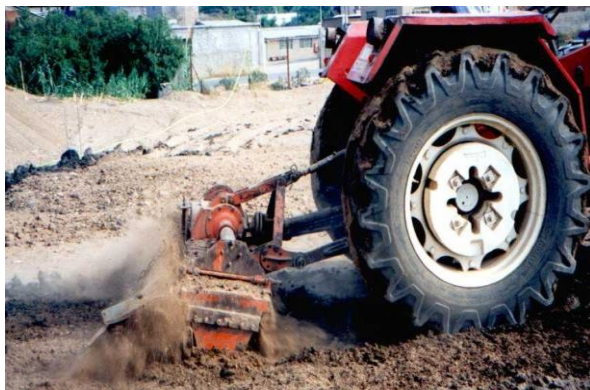
Photo 33. Mixing of the flotation tailings with stabilisers.
