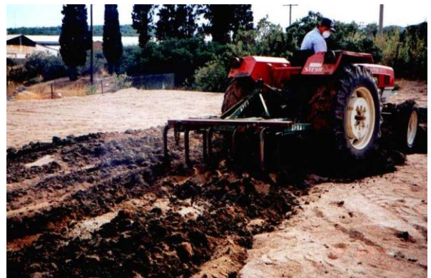
Photo 33. Mixing of the flotation tailings with stabilisers.
