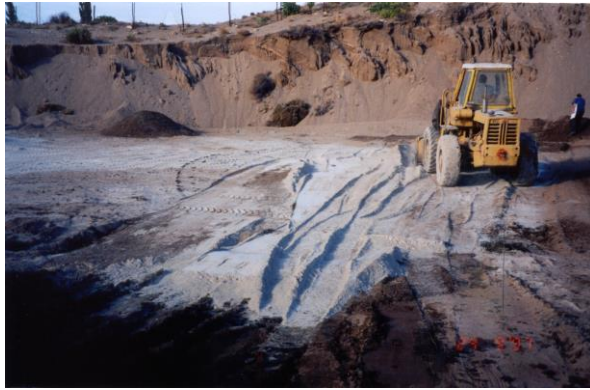
Photo 31. Laying down of fly ash.
