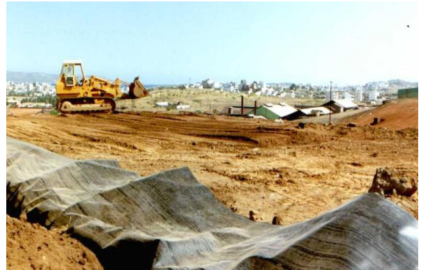
Photo 9. Installation of vertical geomembrane liners for the isolation of test plot areas.
