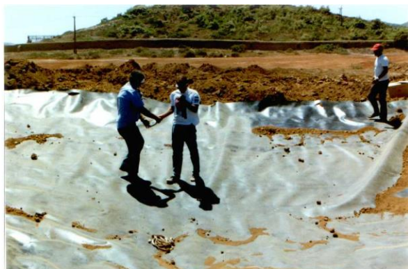
Photo 11. The installation of water collection system at the bottom of lysimeters.
