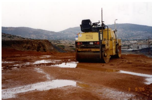
Photo 17. Compacted Clay Cover. Compaction of the clay layer.
