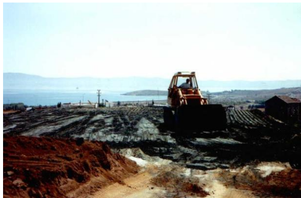
Photos 19. The deposition of Bodosakis pyrites at the Kavodokanos test area.
