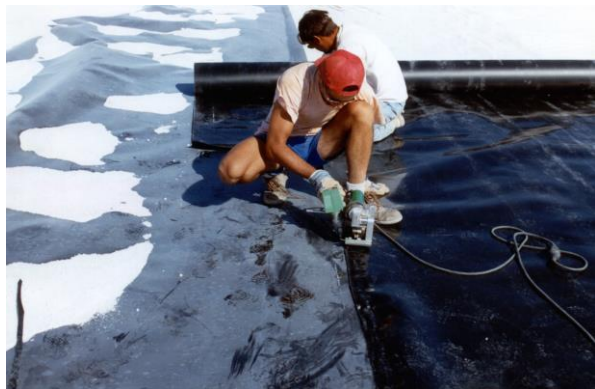
Photo 15. HDPE Cover. Welding of geomembrane sheets.
