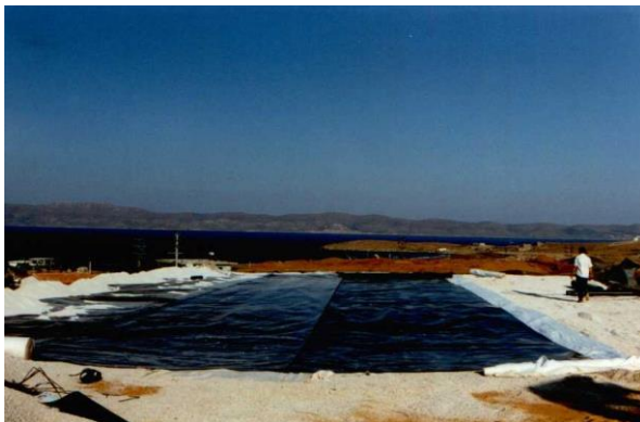
Photo 14. HDPE Cover. The geomembrane liner.
