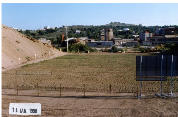
Photo 38. Overview of the area (Jan. 1998).
