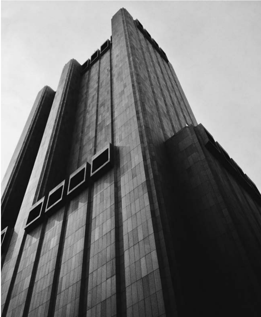
3.12a Long Lines Building, John Carl Warnecke, Manhattan, NY (1969-1974).
