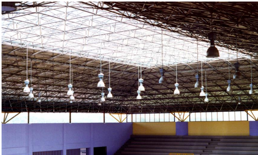
Figure 10: b. Double layer - UABJ Arena in Oaxaca, Mexico
