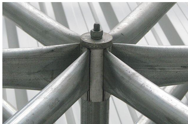
Figure 29: Photo of triodetic node
