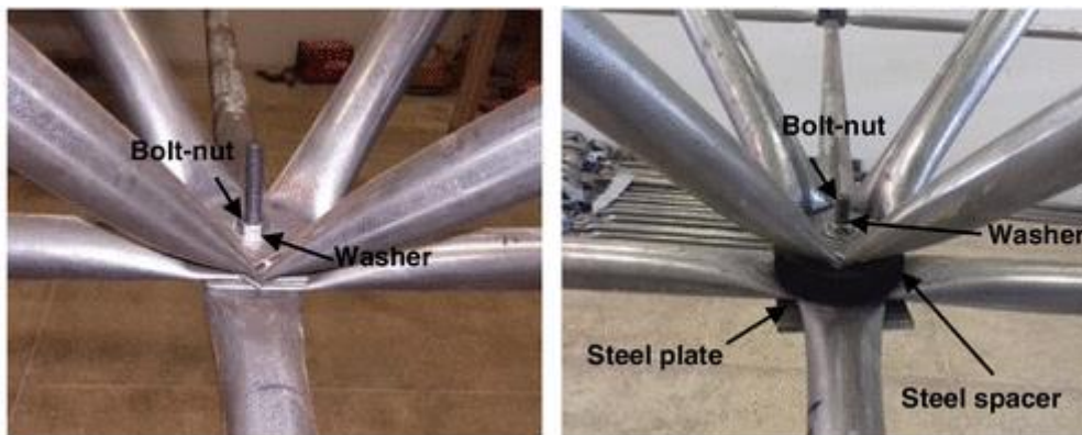
Figure 33: Steel spacer
