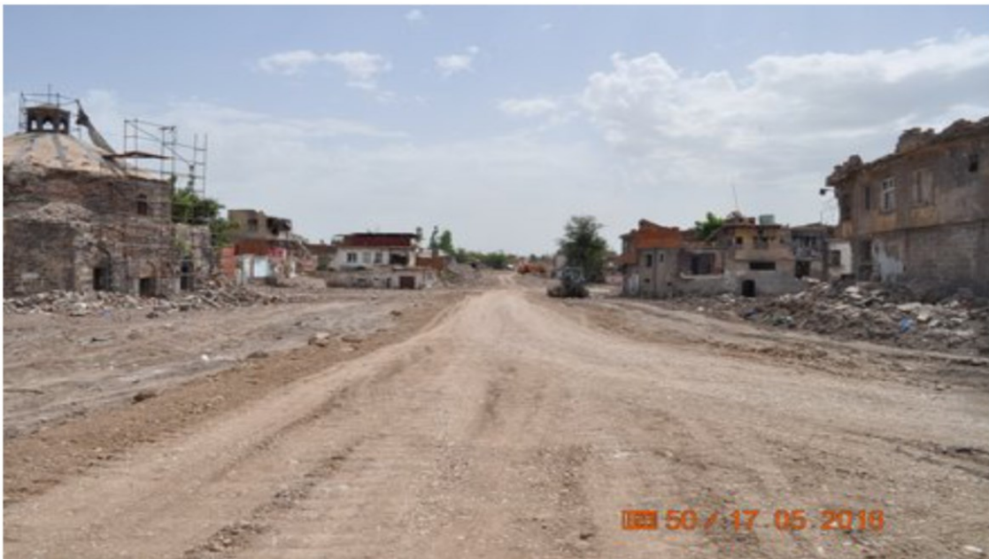
Figure 8.13. Yenikapı Street during street demolition and widening (Soyukaya, 2017, p. 6).
