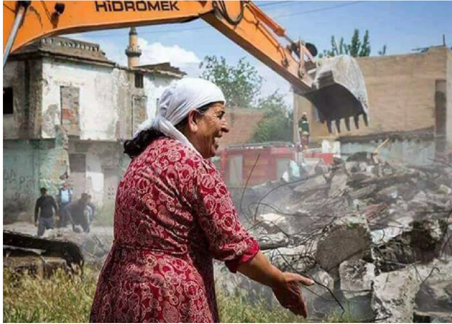
Figure 7.31. Demolitions, Alipaşa and Lalebey (TMMOB, 2019, p. 76).
