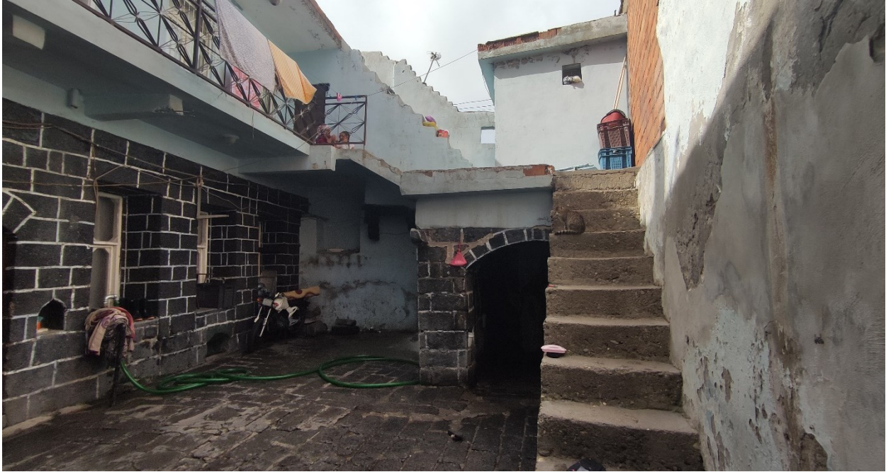
Figure 5.24. Multi-family residence house, with an inner courtyard and newer additions (taken by the author, 2022).
