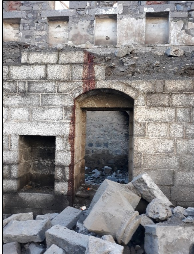
Figure 7.6. Inside the ruined Surp Sarkis Armenian church showing blood reported to be from a thief injured while removing historical stones (Aydın et al., 2020, p. 17).
