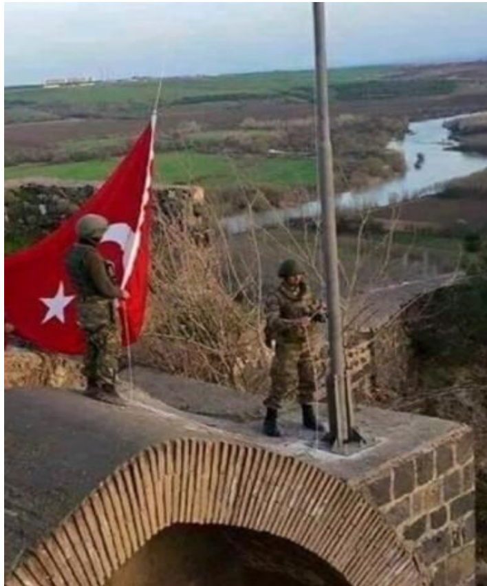
Figure 9.13. Damage done to the historical walls to install a flagpole (DBB, 2016a).
