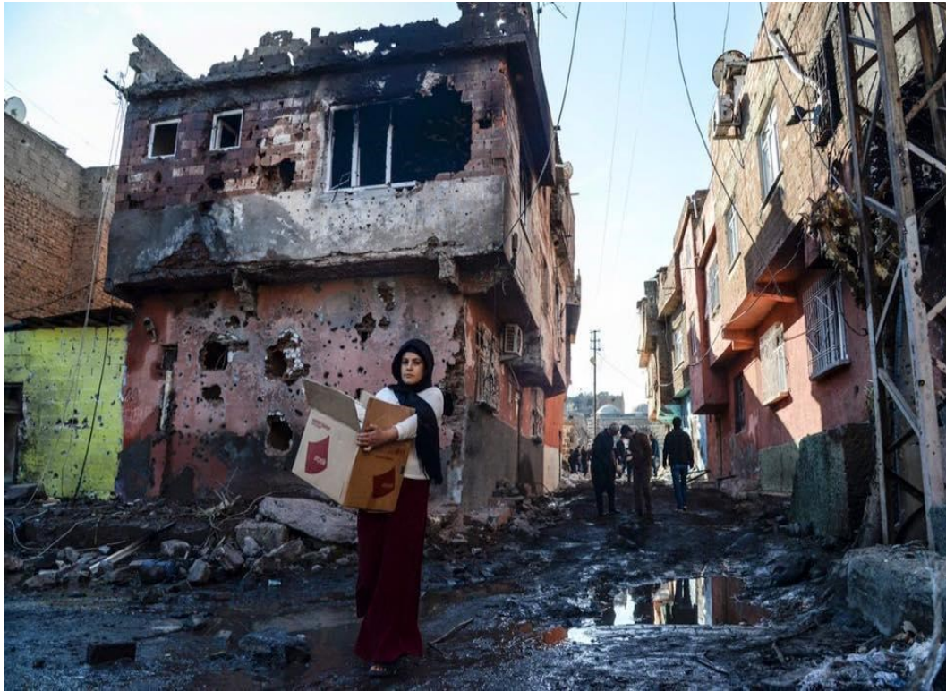
Figure 7.29. Displacement and damaged houses (ROAR collective, 2015).
