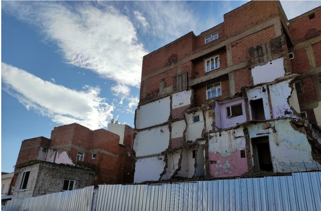
Figure 7.3. Part-demolished area in Sur (taken by the author, 2022).
