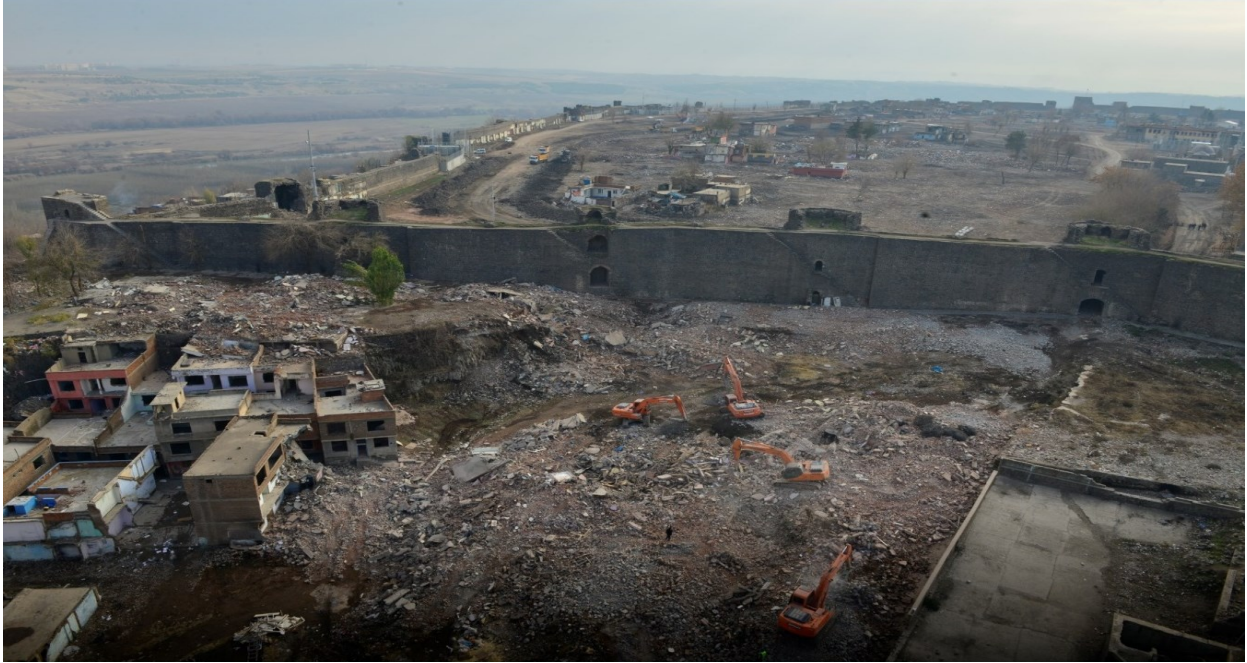
Figure 5.40. Demolition in İçkale (ÇŞİDB, 2017).
