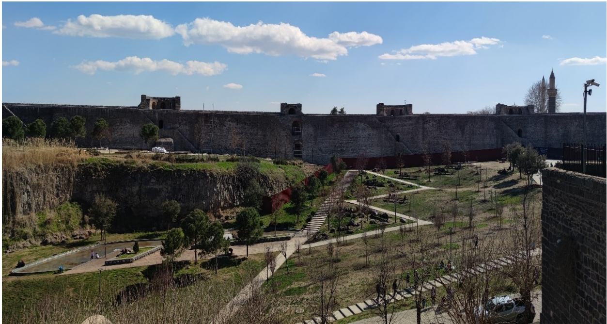
Figure 5.41. İçkale after the demolition (taken by the author, 2022).
