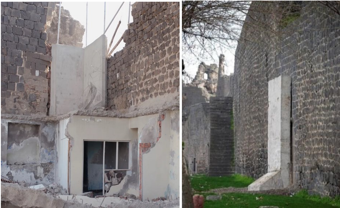
Figure 7.7. Damage to the historical walls with fortification and concrete constructions (left: 140 jounos, 2017; right: DBB, 2016a).
