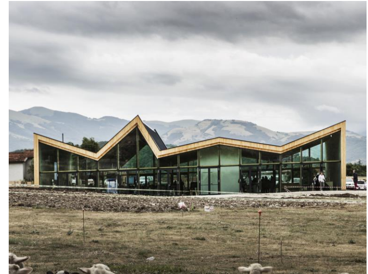
Multipurpose and Civil Protection Center of Norcia / Stefano Boeri Architetti
