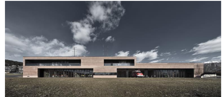
Civil Protection Centre Ritten / Roland Baldi Architects
