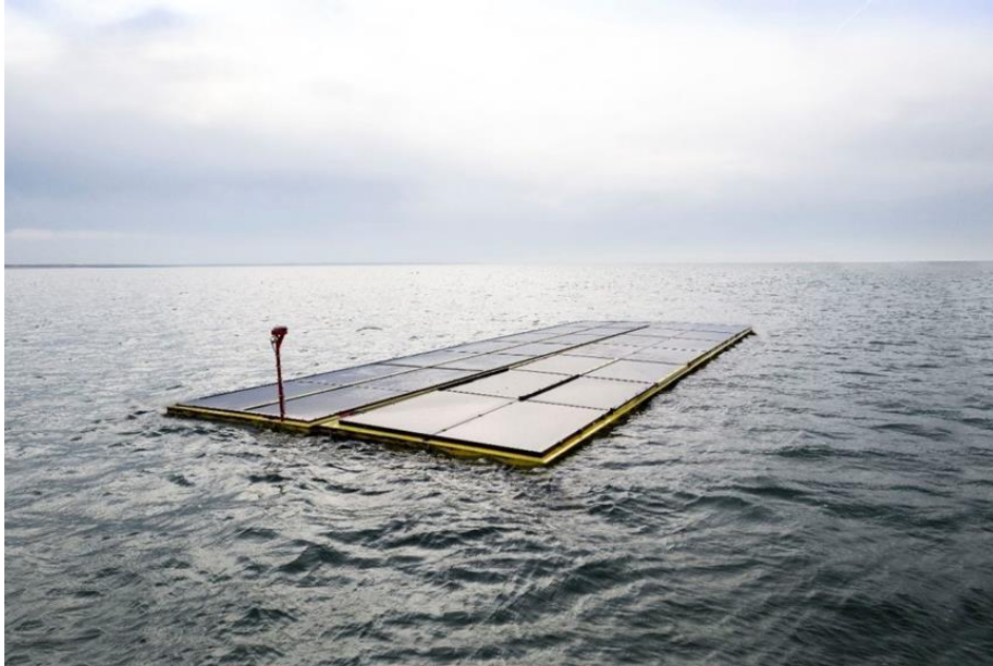
Figure 3. Offshore floating photovoltaic (FPV); (Source:[23])
