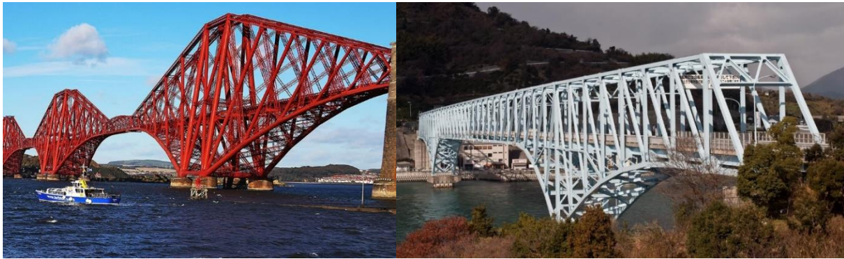
Σχήμα 1.11 Forth Bridge Queensferry, Scotland (1890) & Kamagari Bridge, Hiroshima, Japan (1979).
