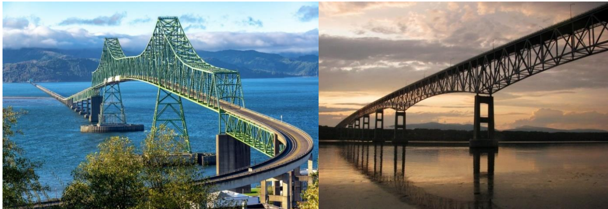
Σχήμα 1.12 Astoria Megler Bridge, Oregon, USA (1966) & Kingston-Rhinecliff Bridge, New York (1957)
