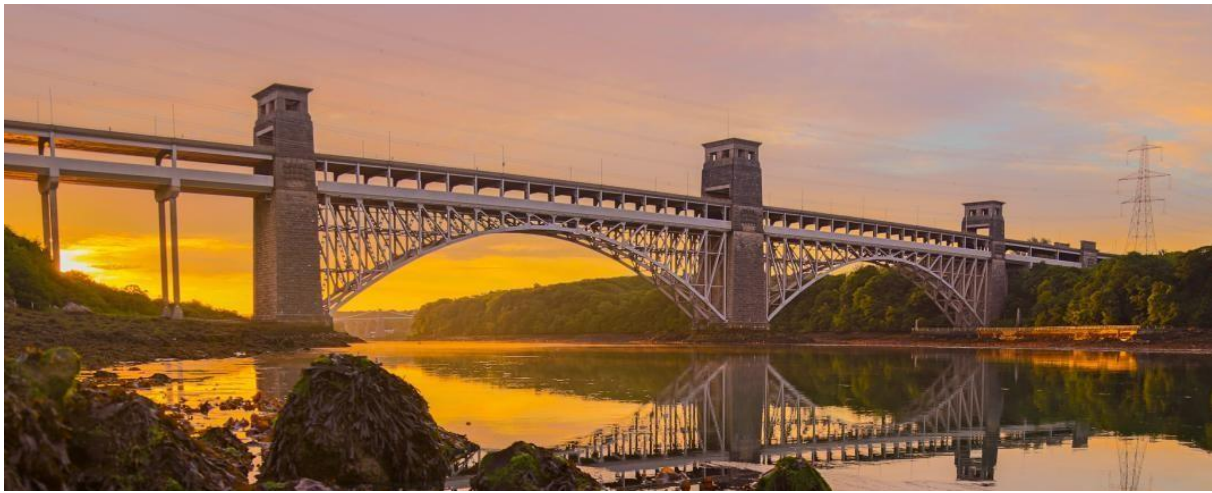
Σχήμα 1.16 Britannia Bridge, Anglesey, North Wales (1980)
