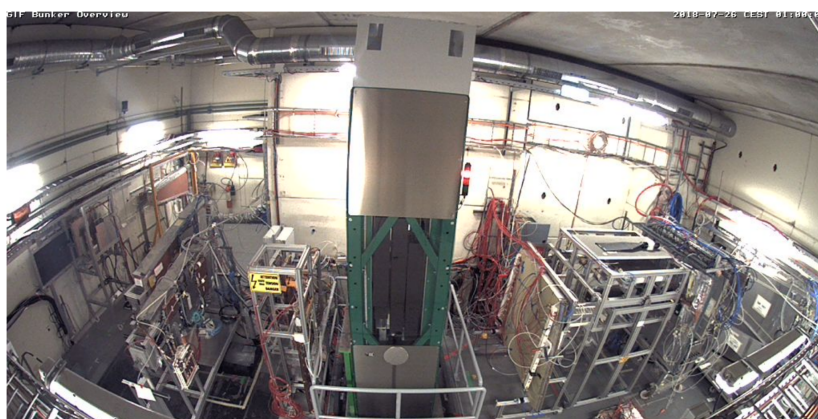
Figure 5.32: The SM2 MM module in the GIF++ facility, facing the source.
