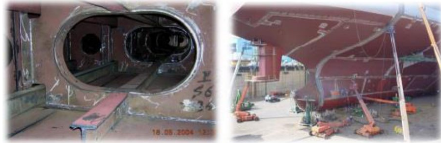
Figure 37: Photos taken during the “secondary” surface treatment (PST, Photo Gallery, 2015)
