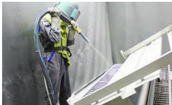
Figure 5: Example of the blast-cleaning method depicted (Hempel, Guideline for Corrosion Protection, 2019)
