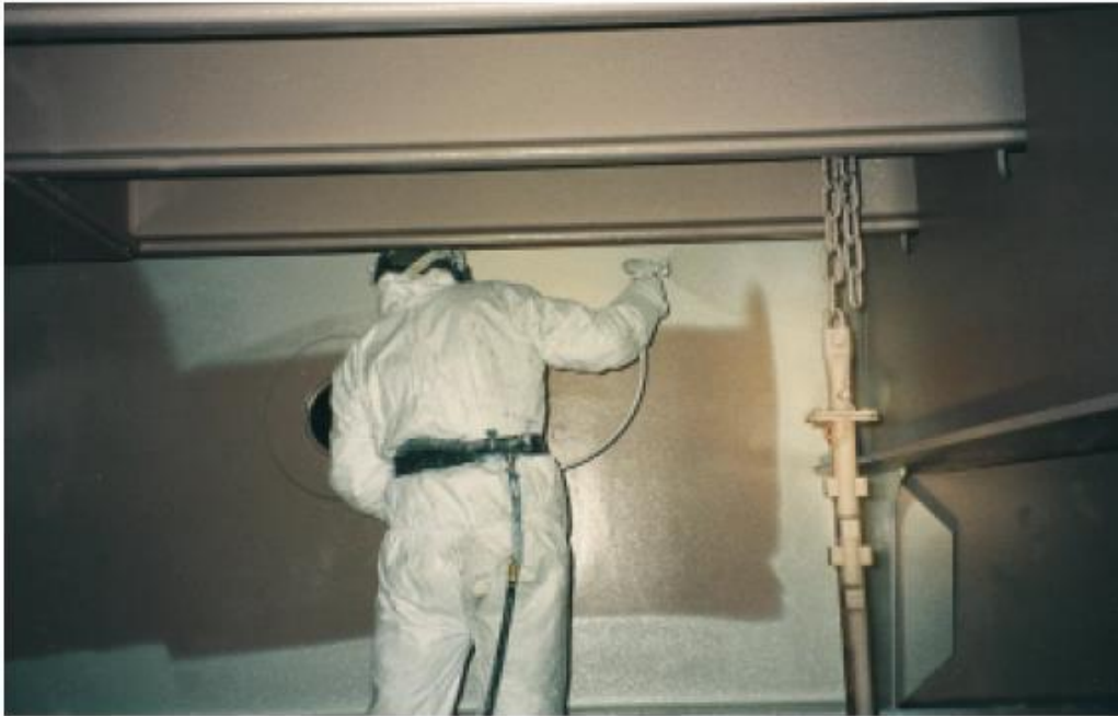
Figure 2: Light colors in dark areas assist application and inspection, (PST Photo Gallery, 2015)
