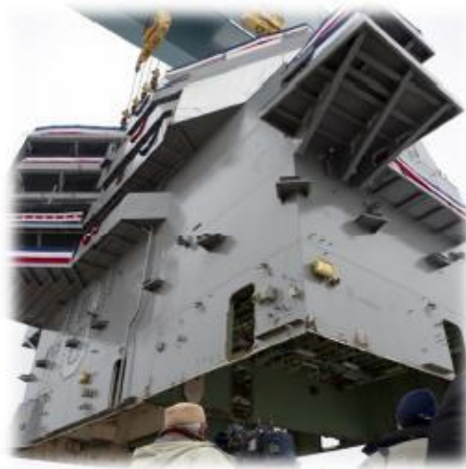
Figure 56: Superstructure (PST, Photo Gallery, 2015)
