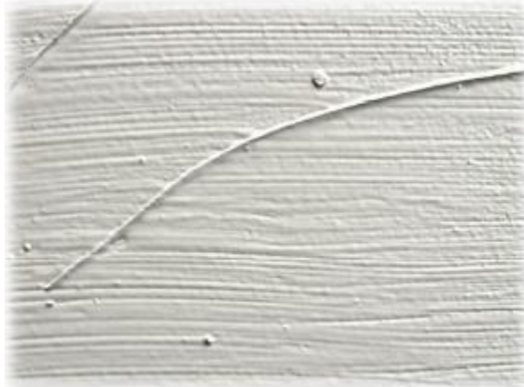
Figure 62: A hair of brush, causing the defect (Coating Manual, Jotun, 2018)
