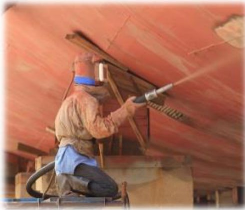
Figure 43: Dry abrasive blast-cleaning (PST, Photo Gallery, 2015) Figure 44: Wet abrasive blast-cleaning (PST, Photo Gallery, 2015)
