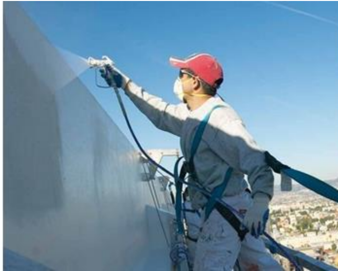
Figure 48: Applying paint with the use of airless spray (PST, Photo Gallery, 2015)
