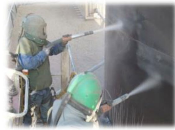
Figure 43: Dry abrasive blast-cleaning (PST, Photo Gallery, 2015) Figure 44: Wet abrasive blast-cleaning (PST, Photo Gallery, 2015)
