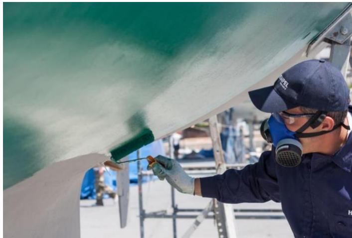
Figure 47: Paint application by roller (PST, Photo Gallery, 2015)
