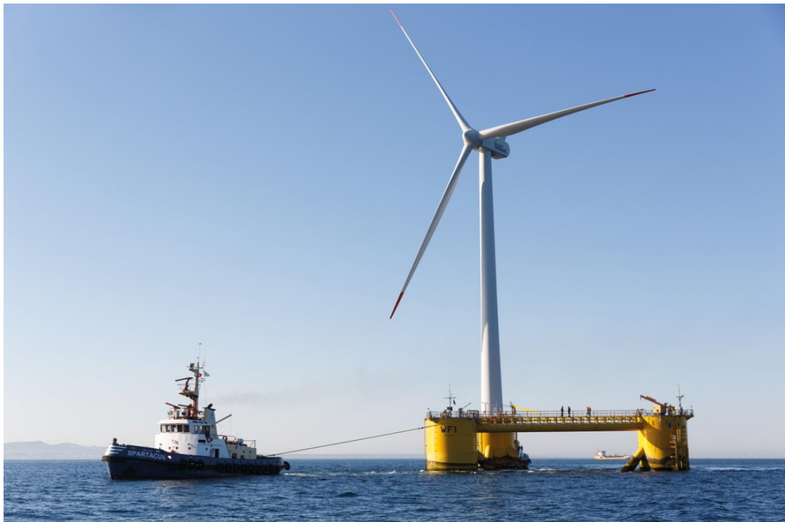
Figure 1. Offshore Wind Turbine (Source: Wind Europe)
