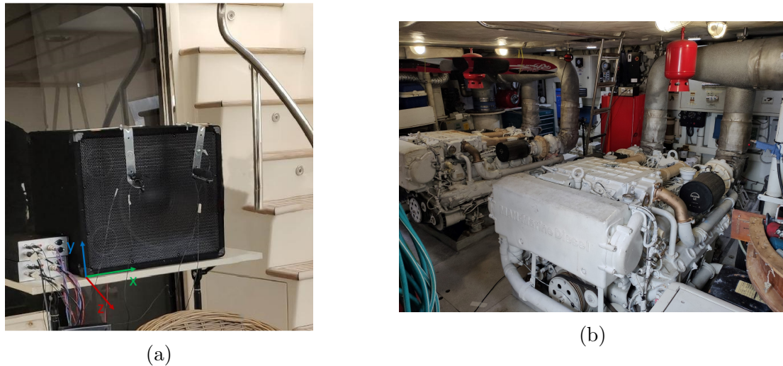
Figure 3.10: a) The active headrest system implemented on the yachts deck, b) the engine room, with two electric generators (ONAN 17 KW), where the reference microphone was placed.
