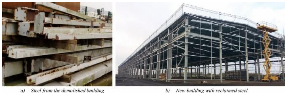
a) Steel from the demolished building
