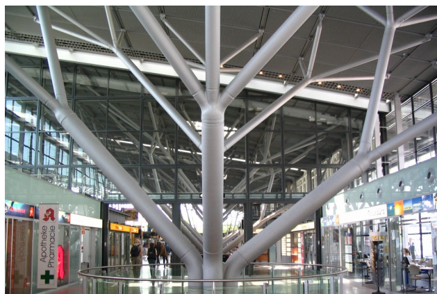
Εικόνα 6_13: Stuttgart Airport terminal, λεπτομέρεια υποστηλώματος Πηγή: Stuttgart Airport Interior 2005-06-02.jpg, Image of the interior of Stuttgart Airport (between Terminal 1 and 3) taken on 2005-06-02 by James Bowes., https://commons.wikimedia.org/wiki/File:Stuttgart_Airport_Interior_2005-06-02.jpg , εικόνα του/της: No machine-readable author provided. JamesBowes assumed (based on copyright claims), άδεια: CC BY-SA 3.0, Creative Commons Attribution-Share Alike 3.0 Unported license.
