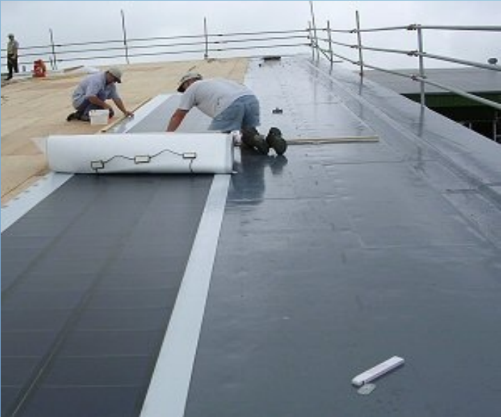
PLACING PHOTOVOLTAIC ELEMENTS on a roof [photovolt. waterproofing membranes]
