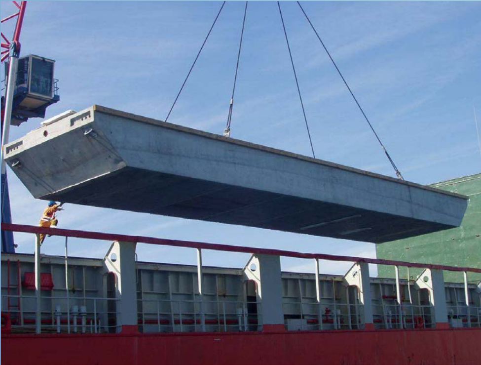
Part of floating breakwater
