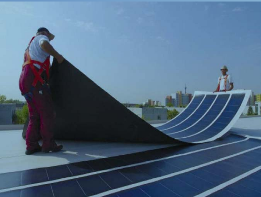
PLACING PHOTOVOLTAIC ELEMENTS on a roof [photovolt. waterproofing membranes]
