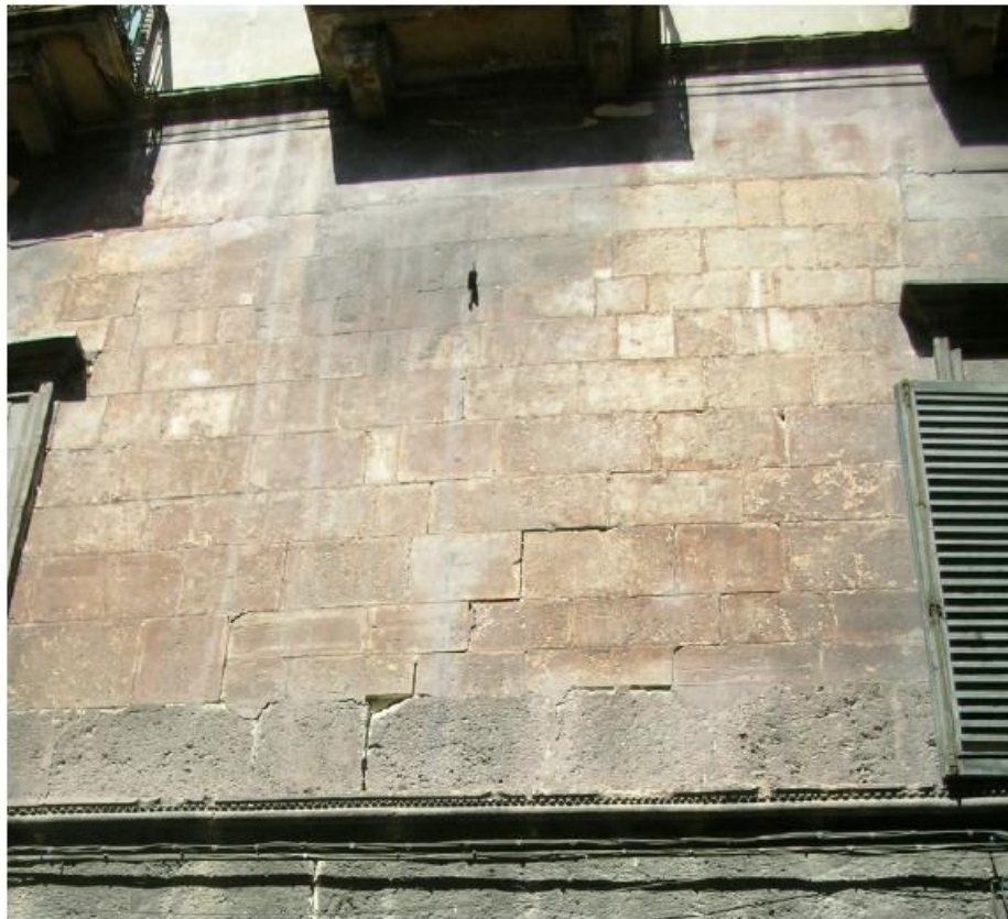
Fig. 12 Shear failure of masonry (from E. Vintzilaiou – “Lecture notes on Advanced Mechanics of Masonry”)
