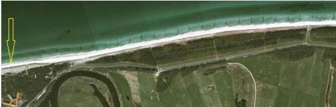
Figure 2.9: Left part of the groyne system (source: Google Earth)
