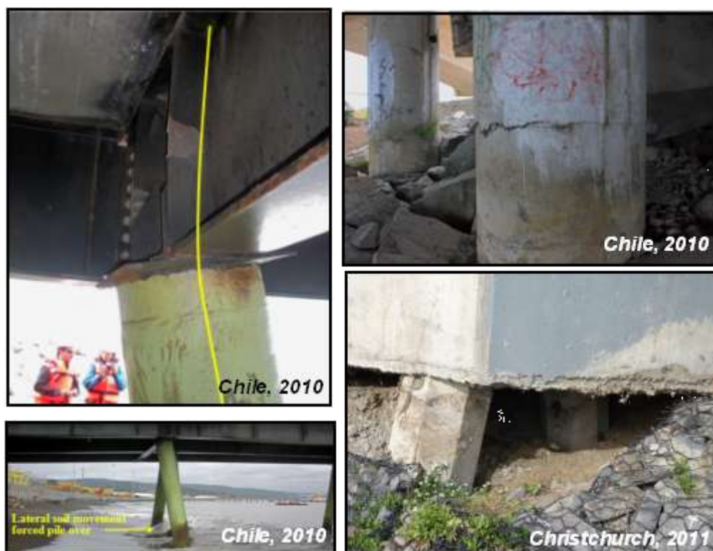
Figure 1.3: Pile failure due to liquefaction-induced lateral spreading from the Chile, 2010, M=8.8 and the Christchurch, New Zealand, 2011, M=6.3 earthquakes.
