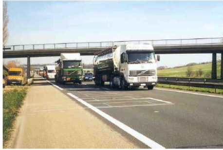
Picture of Metz MS-WIM array, A31, France
