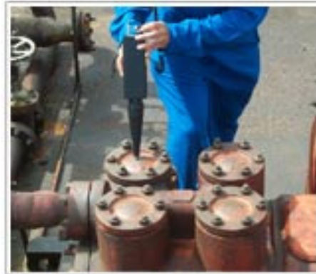
Airborne Ultrasound Mechanical Inspection
