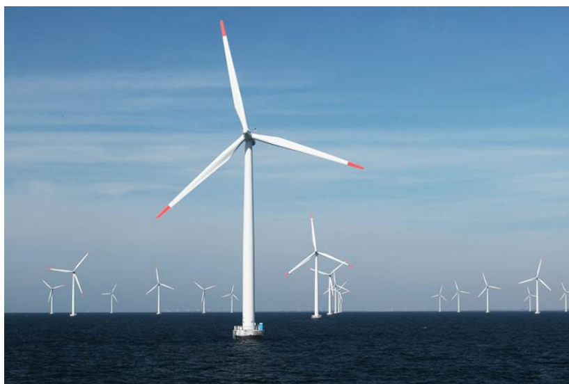
London Array offshore wind park
