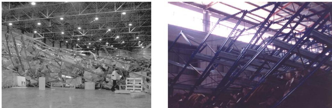
Figure 1.3: The "Domino-effect" collapse
