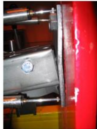
Base bending and weld failure
