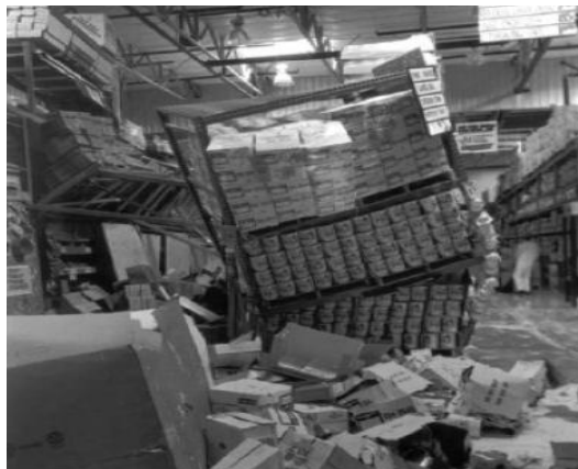
Figure 1.2: Cross-aisle collapse
