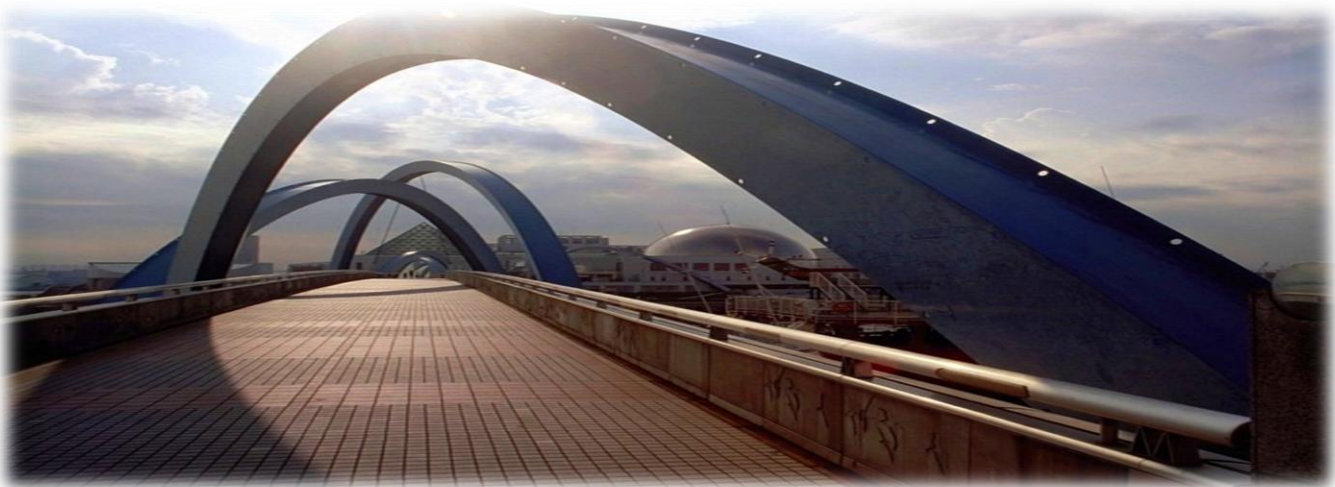
Nagoya Pedestrian Bridge
