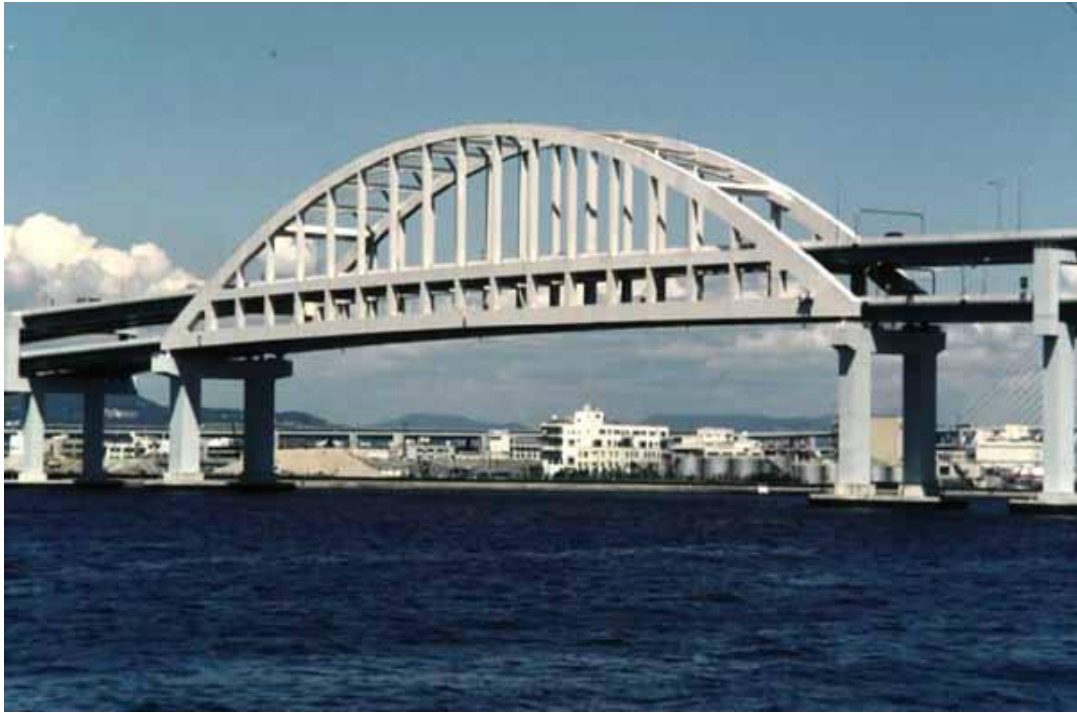
Figure 1.3 The Nishinomiya-ko bridge in Kobe, Japan
