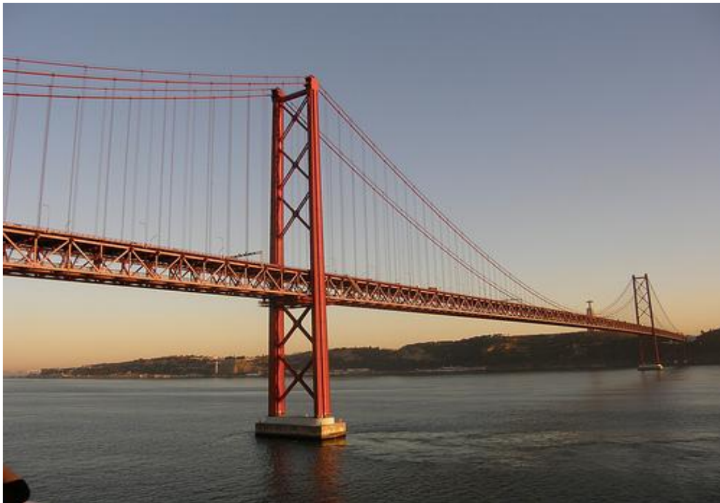
Figure 1.2 The Tagus River Bridge in Portugal, founded on a 88 – m high caisson.
