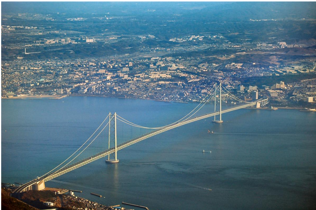
Figure 1.4 The Akashi-kaikyo bridge in Kobe, Japan founded on two massive 80-m diameter caissons.
