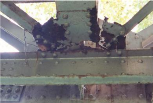
Figure 23 : Bridge Corrosion
