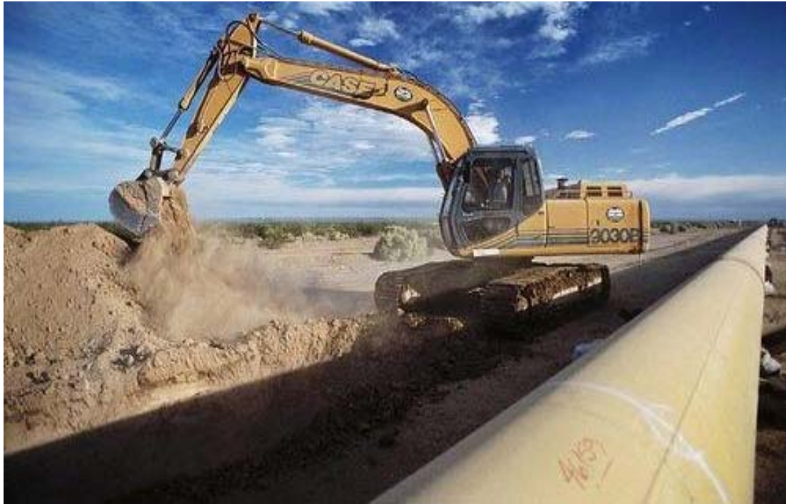
Figure 1.3.2. Excavation of the trench ( www.constructionphotography.com ).
