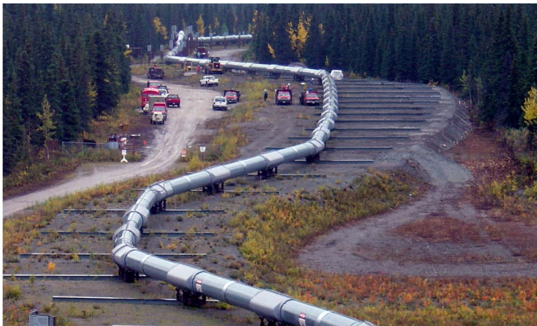
Figure 1.3.1. The trans-Alaska oil pipeline where it crosses the Denali Fault. The special footings allow the pipe to move 6m laterally and 1.5m vertically (Alaska Natural Gas Transportation Projects).
